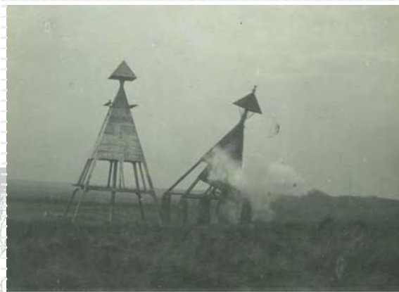
Demolition of Donna Nook Beacon
