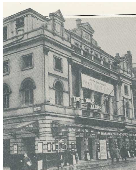
Shaftesbury Theatre (the original) 1939
