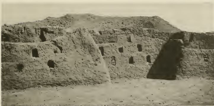
2. BUTTRESS SHOWING ROUGHNESS OF WORK.
