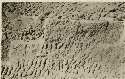
2. PORTION OF A WALL SHOWING BRICKS LAID ON EDGE.
