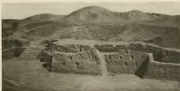
1. BUTTRESS AGAINST FAÇADE OF PALACE.
