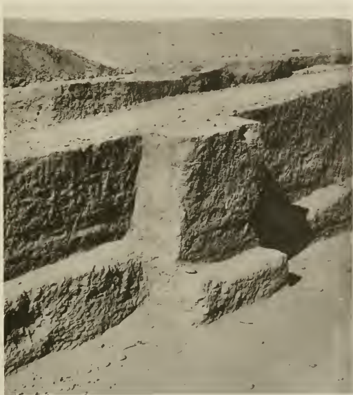
1. BUTTRESS INSIDE OUTER WALL OF ANNEX.
