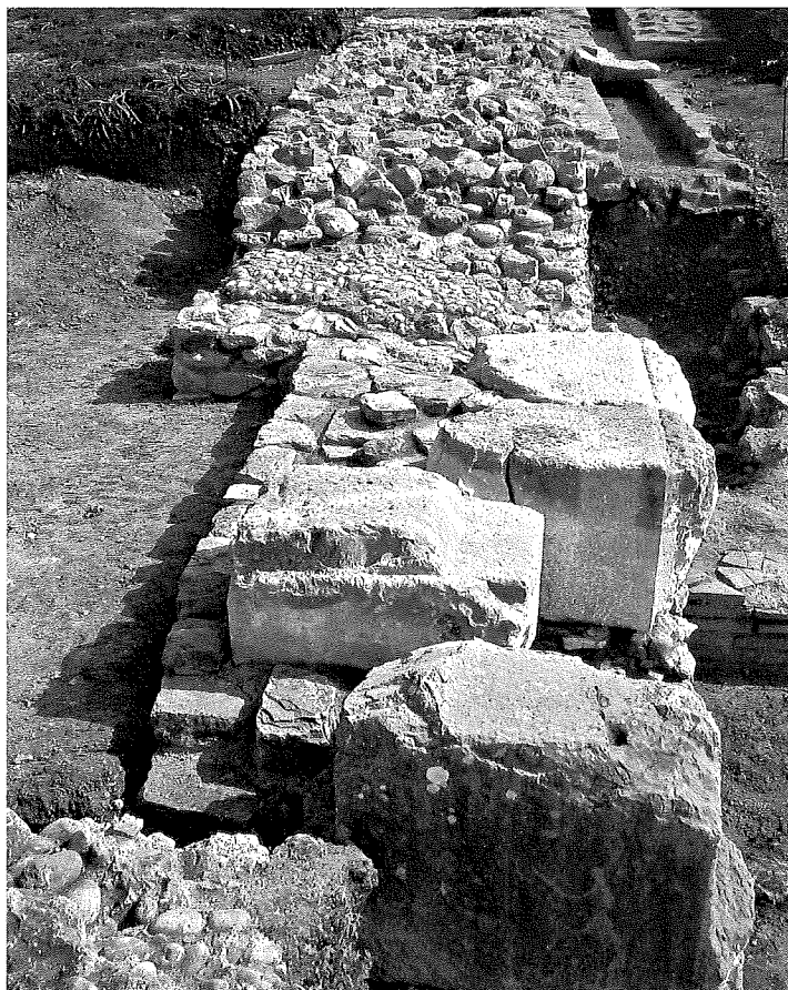
Fig. 10. The E part of the façade retaining wall during excavation.
