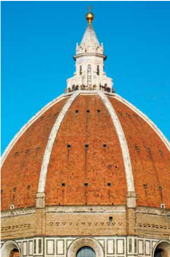
Fig. 2 The 22 m high lantern was completed by Michelozzo in 1461, and the 8 tonne gilded copper ball was added by Verrocchio and Leonardo da Vinci in 1469.
