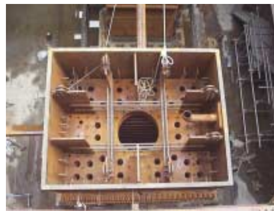
View of super-column shell. At the base, the super-columns are 2.4 m by 3.0 m (approximately 8' by 10').
