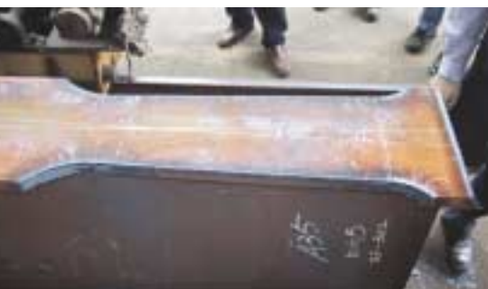
Above and below: At locations where plastic rotation would exceed 0.005 radian in a 950-year return period earthquake, reduced beam sections ("dogbone" cuts) increase moment connection rotational capabilities.
