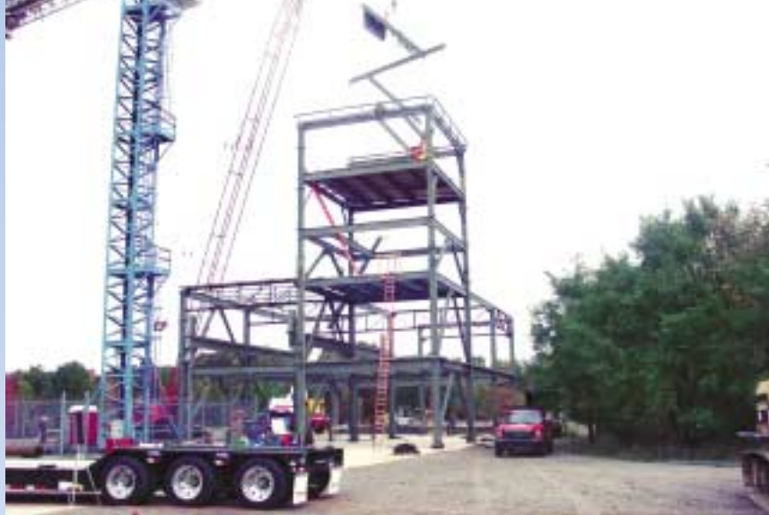
Erectors learn how to safely perform multiple-lift rigging techniques, also known as “Christmas-treeing.”
