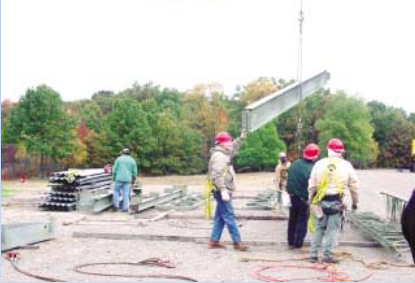
Apprentices get practice in beam-picking procedures.
