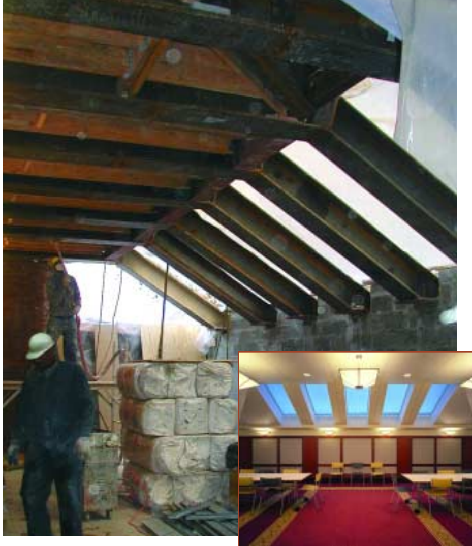
Above: New steel framing supports five floors above—and a masonry bearing wall—to provide column-free space and skylights for the new ground floor Commons Room ( inset ).
