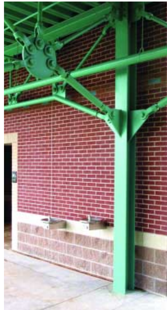
Above and below, right: Structural details using clevises, threaded rods, pipe sections, and plates serve as functional architectural elements.
