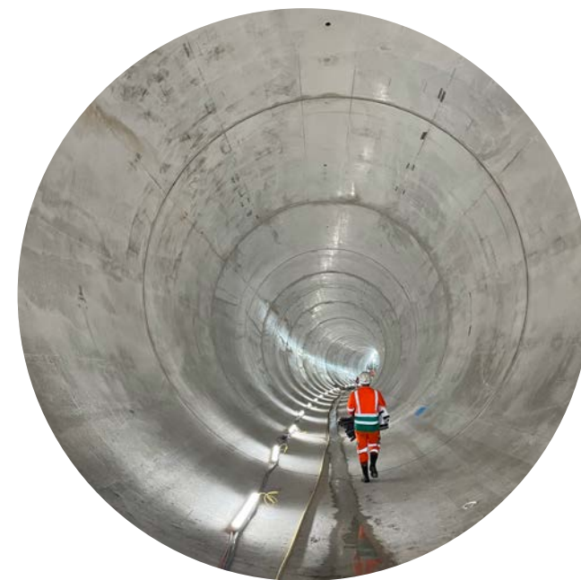
Above: An inside view of the Thames Tideway Tunnel, London's 'super sewer', due to be completed in 2025. Image credit: Courtesy of Tideway.
