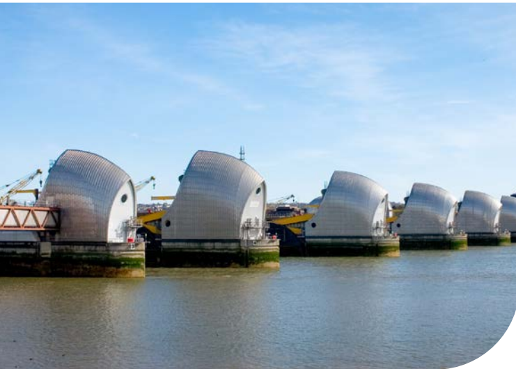
Above: The Thames Barrier, in operation since 1982, helps protect London from flooding.
