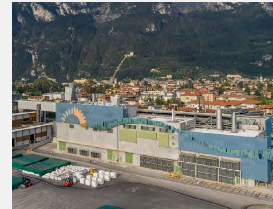
Alto Garda Power plant, Italy
