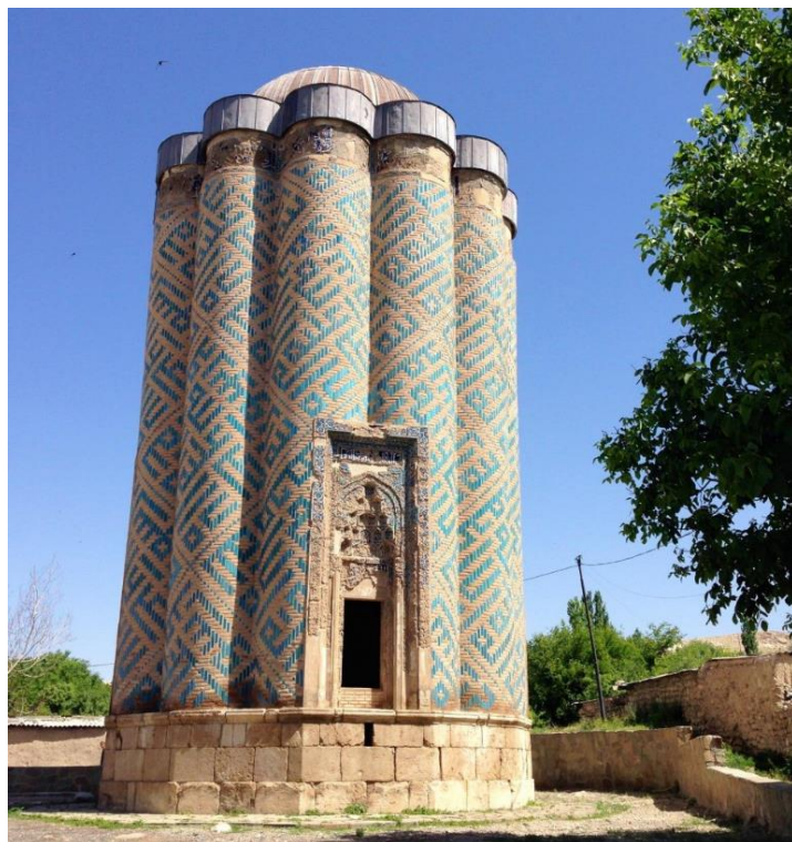
Figure 5.27 Mausoleum in Qarabaghlar village, Nakhchivan which has a dedication to Goday Khatun and probably built during the reign of Abu Said (1316-35) (photo: Kyle Olson, 2014, used with permission)
