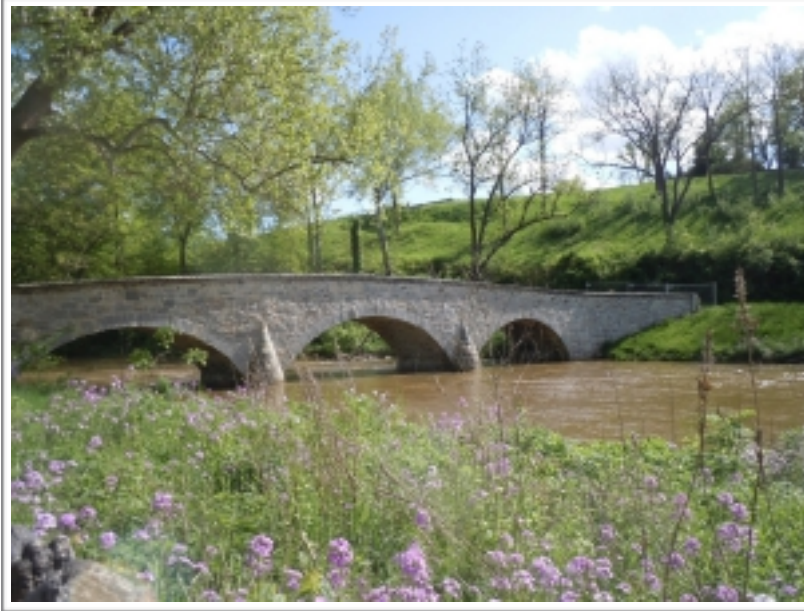
Antietam Creek Bridge (AH)
