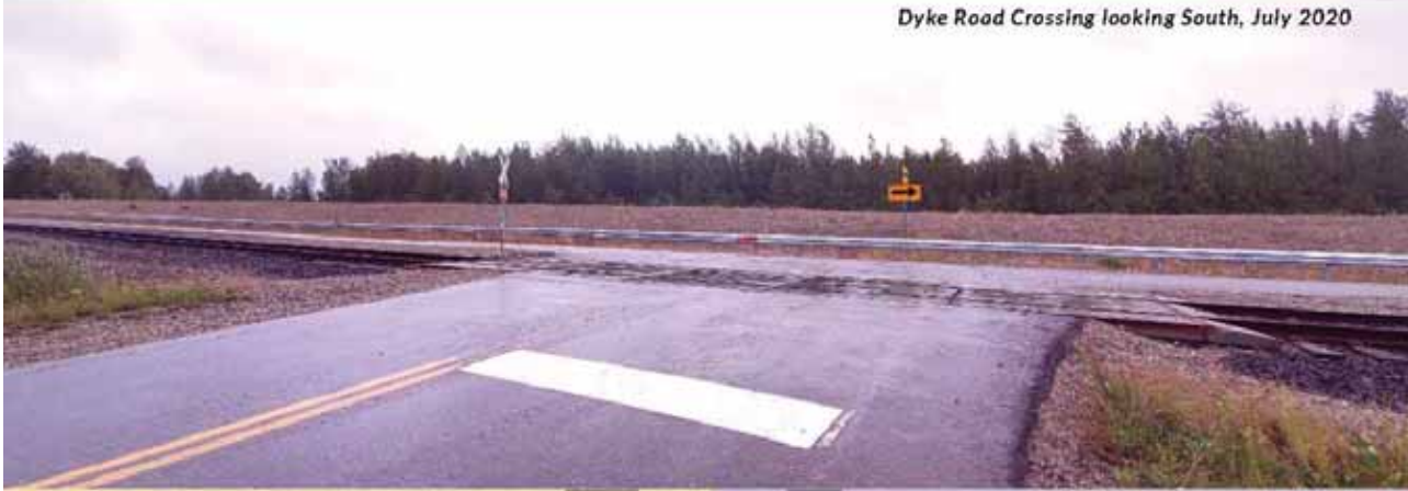
Dyke Road Crossing looking South, July 2020
