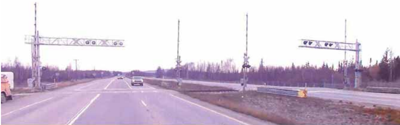
Richardson Highway (3 Mile) Crossing looking Southeast, Google Earth
