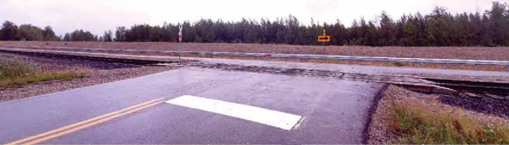
Dyke Road Crossing looking South, July 2020
