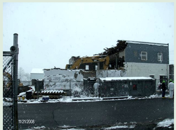
Ron's Rental Demolition
