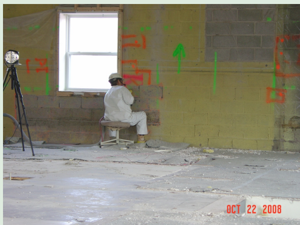
Ron's Rental Interior Radiation Contamination Demolition
