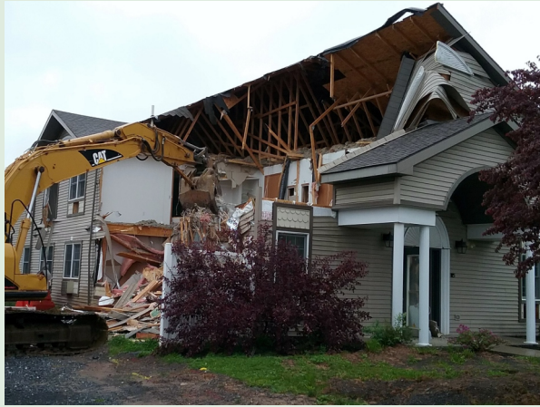
Former Lock Haven Court Demolition
