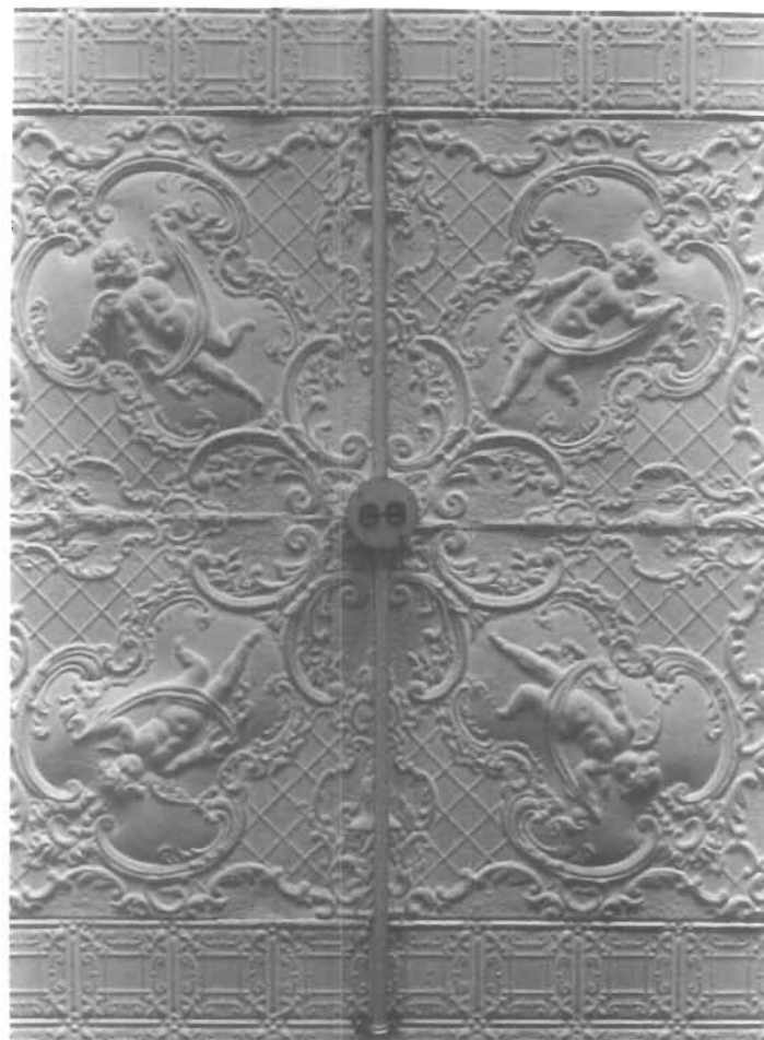
Figure 101. Pressed Metal Ceiling, 212 West Main Street, Johnstown, New York. Mistakenly called "tin ceilings," pressed metal ceilings were stamped sheet iron and later sheet steel; only one or two isolated companies coated them with tin. Pressed metal was sometimes galvanized with zinc, especially when used outdoors or as porch ceilings. It was sold by the sheet with the patterns fitting neatly together for covering ceilings and sometimes walls or wainscoting. Accessory pieces, such as ceiling medallions, were available. Cornices provided the transition from ceiling to walls. (Becket Logan)
