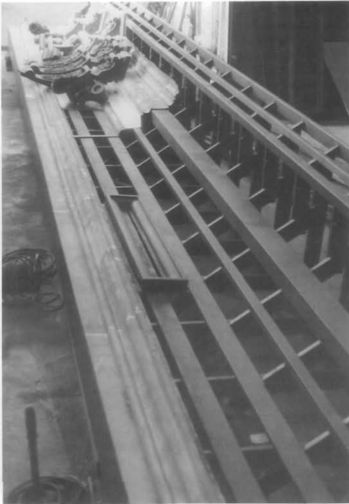
Figure 143. Preassembling Cornice. As illustrated in figure 142, most sheet-metal cornices were supported by wooden support members projecting out from the facade of the building either as an extension of the roof framing or as a cantilever from a parapet wall. In either case, these wooden support members are often found to be rotten and have to be replaced. For large cornices high above the street level, it may be economically unfeasible to use scaffolding for in situ repairs and reconstruction unless the scaffolding is also needed for other work. The entire galvanized sheet-iron cornice of the ZCMI Store in Salt Lake City, Utah, was pre-assembled on the ground with repaired original parts and some new pieces onto a new support system fabricated on small steel angles. Fifty-foot sections of the preassembled cornice were then hoisted to the top of the facade and bolted onto the building without the need for scaffolding. (Steven T. Baird)
