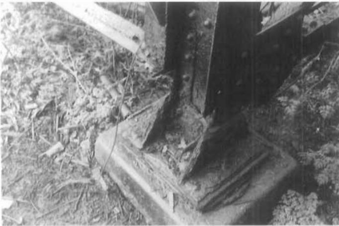
Figure 158. Advanced Corrosion of Rolled Iron. This column base of a New York Central Railroad pedestrian overpass has not been well maintained and has rusted beyond repair. Such exposed ironwork should be painted regularly to keep it from contact with air and moisture. Note the characteristic way that wrought-iron rust exfoliates, or flakes off in layers. (John G. Waite)
