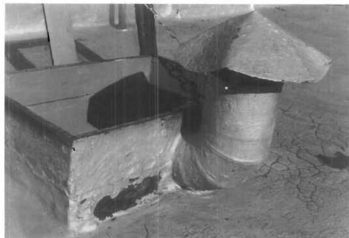
Figure 128. Deterioration of Tinplate by Asphalt Coating. The tinplate flashing of the roof hatch has been corroded away (between the corner and the vent) by the action of the asphalt coating and water. (John G. Waite)
