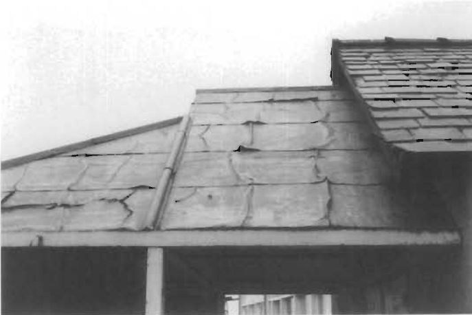
Figure 119. Creep. Deterioration of milled sheet lead roof on a 19th century canal warehouse and office at Nantwich Basin of the Shropshire Union Canal at Nantwich, Cheshire, England. The failure has been caused by creep and the expansion and contraction of the lead. (John G. Waite)
