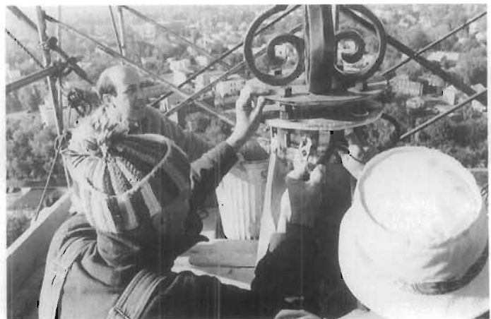
Figure 177. Reinforced Polyester Replica. The original cross of St. Agnes Church, Cohoes, New York, was removed from the steeple in the 1890s to serve as a grave marker. The original wrought-iron steeple cross, still intact, was used as a model to cast a new cross of reinforced (fiberglass) polyester. Fiberglass was chosen as a substitute material because of the inaccessible location (top of the steeple) where maintaining wrought iron (painting) would be difficult and expensive and because from the street level no one would be able to detect the substitute materials. (John G. Waite)
