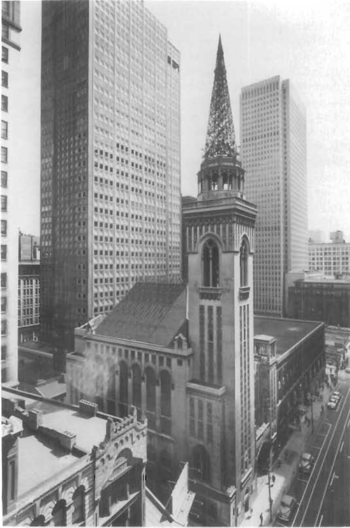
Figure 113. Cast Aluminum Spire, German Evangelical Protestant Church, Pittsburgh, Pennsylvania, 1926; Henry Hornbostel, architect. Also Alcoa Building (background, left), Golden Triangle, 1952; Harrison and Abramovitz, architects. The perforated spire of the German Evangelical Protestant Church, now the Smithfield Street Congregational Church, consists of 22 filigree aluminum castings. The Alcoa Building is the first multistory structure with an aluminum curtain wall. The other tall building (right) is the United States Steel-Mellon Building. (Carnegie Library of Pittsburgh)
