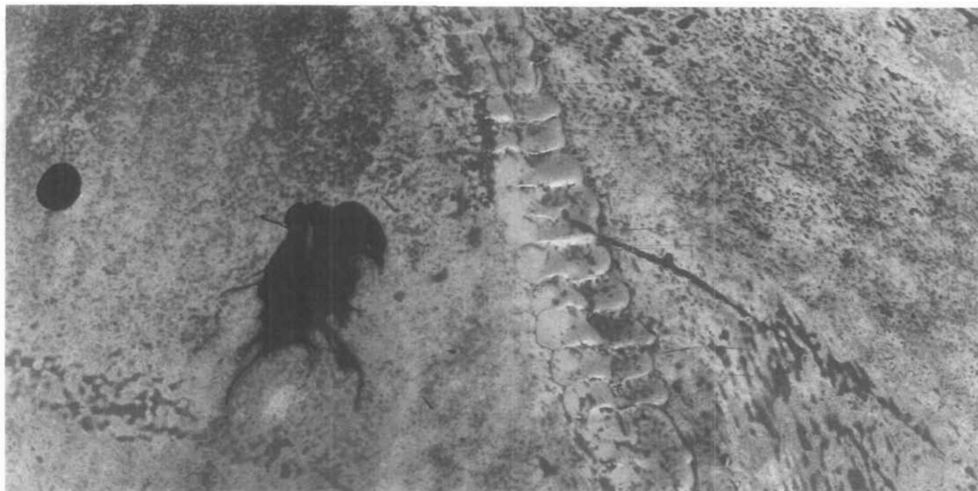
Figure 130. Modern Solder Joint on a Terneplate Roof. Solder was used to make watertight joints at the edges of terneplates on flat-seam roofs. Nineteenth-century soldered joints were almost invisible, that is, the solder was confined to the seam. These wide-soldered joints are on the Old Pension Building in Washington, D.C. The problems with wide-soldered joints are: (1) they facilitate galvanic corrosion because they provide a wider surface area with which the plates can react, and (2) they tend to fail because of the different coefficients of expansion and contraction of the solder and the terneplate. The black spots to the right of the solder are asphalt or a bituminous roof patching compound, which may cause deterioration of the terneplate and should be removed. (David W. Look)
