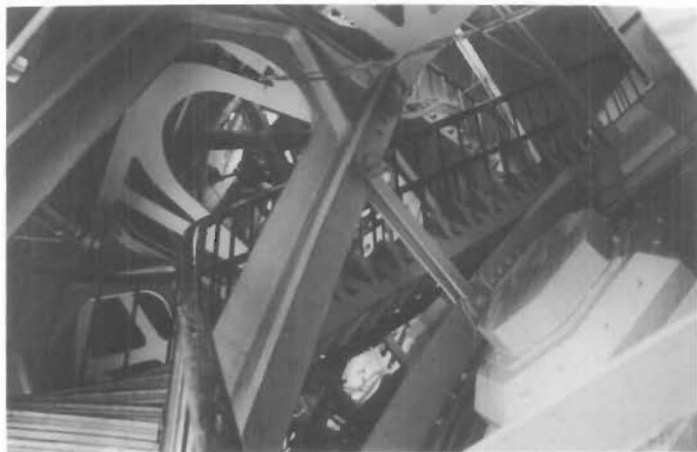
Figure 74. Stairs between the Inner and Outer Domes, U.S. Capitol, 1856–1865; Thomas U. Walter, Architect of the Capitol; Montgomery C. Meigs, engineer. The double shell dome construction is supported by 36 radiating, arched trusses. In this view of the stairs to the lantern, every element is cast iron except the wrought-iron tie rods and bolts. To the right is the back side of one of the cast-iron coffers of the inner dome. The center of the coffer can be unbolted for inspection and maintenance of the inner dome. (David W. Look)
