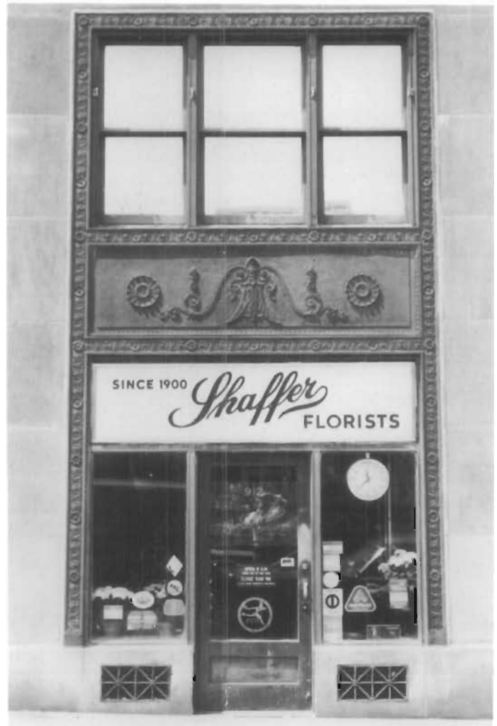
Figure 32. Bronze Storefront, Grilles, Spandrel Panel, and Window, Southern Railway Building, 912 Fifteenth Street, NW, Washington, D.C., 1928; Waddy Butler Wood, architect. This building is typical of many large commercial buildings with extensive use of bronze. Everything from the grilles to the windows and spandrels to the storefronts were fabricated of bronze. Although many storefronts have been remodelled beyond recognition, this one still has its original design and materials. (David W. Look)
