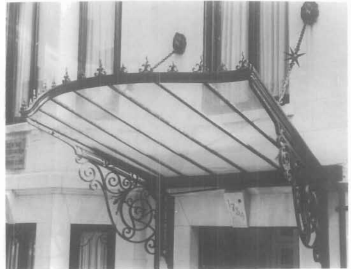
Figure 56. Wrought-iron and Glass Canopy, 1734 N Street, NW, Washington, D.C., ca. 1885. Iron is found in a variety of forms from strap hinges to fragile glass and iron combinations—such as the canopy protecting the entrance of this elegant townhouse. Glass panels were set in an iron frame with fleurs de lis on the front edge and flourishes as supporting brackets. (David W. Look)
