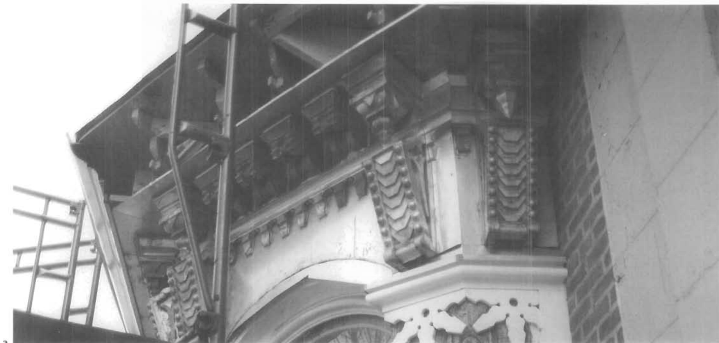
Figure 142. Restoration of Galvanized Sheet Iron and Cast-Zinc Cornice. This is the upper third of a wooden bay window on a Second Empire brick rowhouse in the Logan Circle Historic District of Washington, D.C. (a) From the window down, the bay is wood and glass. The roof of the bay had leaked for years and the wooden roof rafter and projecting supports for the cornice had rotted. The bay window was carefully disassembled and rebuilt replacing all deteriorated lumber. The surviving pieces of galvanized sheet-iron and cast-zinc cornice were taken to a sheet-metal shop. The pieces that were repairable were cleaned; missing portions of brackets on the right were replicated of galvanized sheet iron using the originals as a model. (b) On the opposite side of the bay, all of the brackets and modillions are repaired originals but all of the flat and molded sections are new 26-gauge galvanized steel. The 65-year-old sheet-metal worker on this job said that the only two major advances in metal cornices in his lifetime are the use of pop rivets for fasteners (used also in leatherwork) and the use of autobody putty to patch holes, mold small missing details, and waterproof joints. The putty dries hard and can be sanded. (David W. Look)
