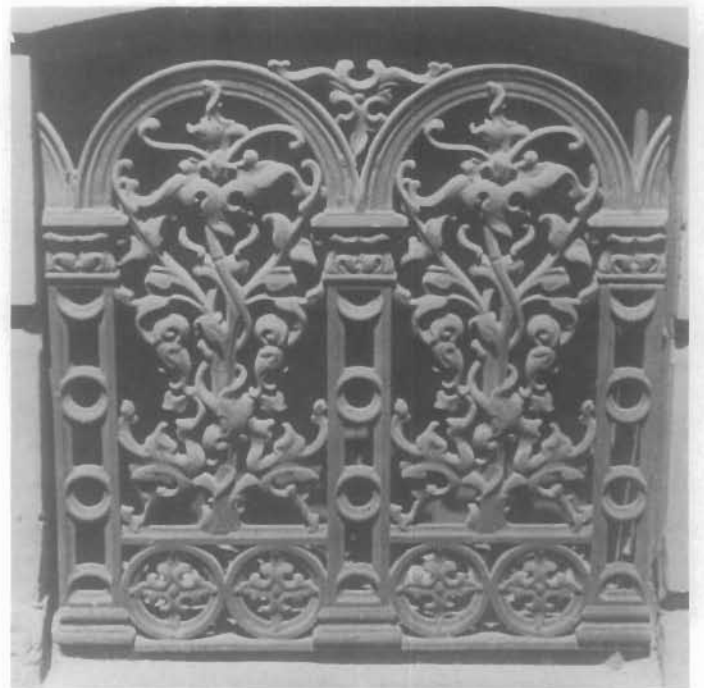
Figure 85. Cast-iron Cellar Window Grille, Matthew Quay House, northeast corner of Spruce and 11th streets, Philadelphia, Pennsylvania. Although little noticed, there is a seemingly endless variety of decorative cellar window grilles in Philadelphia. With the first-floor level several feet above grade and the sidewalks often extending right up to the facade, these articulated iron grilles were installed to protect exposed cellar windows while still allowing ventilation. The grille photographed here displays a motif of cast-iron vines set in a pair of arched panels. (Harley J. McKee, FAIA)
