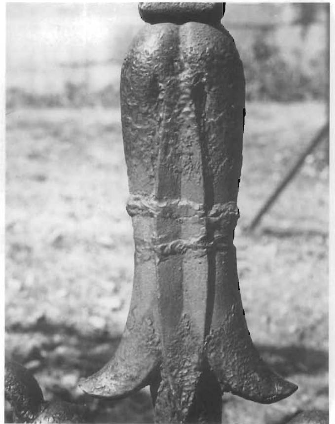
Figure 167. Welding Cast Iron. Although cast iron is very difficult to weld, it can be done by a skilled welder. This is a detail of a weld on the cast-iron fence at the Gardiner-Pingree House in Salem, Massachusetts. "Ni-Rods" welding electrodes, made with a nickel alloy, have been used to weld cast iron since 1947. This weld should have been ground down after completion. (Lee H. Nelson)
