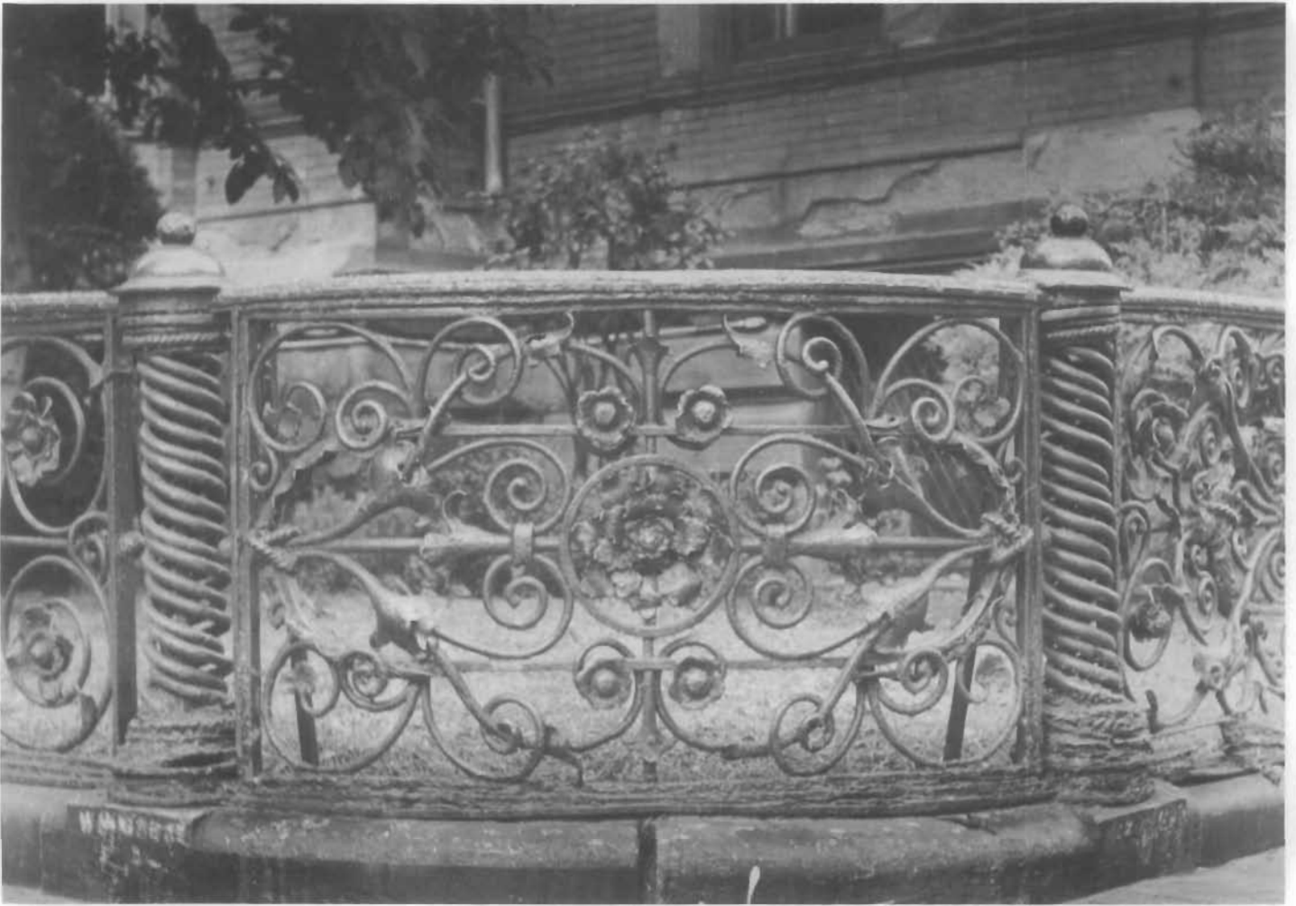
Figure 53. Wrought-iron Fence, Frederick Ames Mansion, 306 Dartmouth, Boston, Massachusetts, 1872; John Sturgis, architect. This fence was fabricated by hand from iron bars; square and round sections were hot-worked into spirals, circles, and scrolls. Even the fence posts are compact spirals of strong rods shaped about a central support to make them rigid. (Esther Mipaaas)
