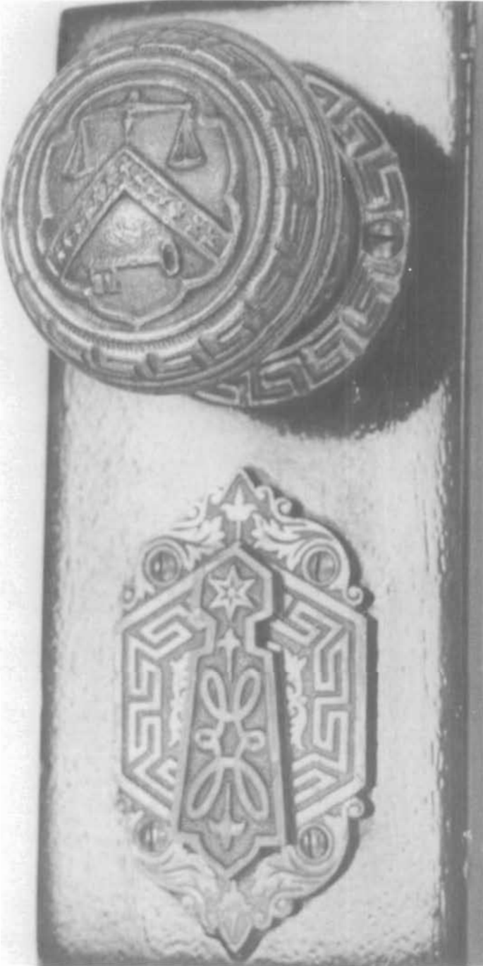
Figure 35. Brass Doorknob and Escutcheon Plate, Old United States Mint, San Francisco, California, 1869-1874; Alfred B. Mullet, architect of the Treasury. Throughout most of the 19th and into the early 20th centuries, hardware was often specially designed for significant public and some private buildings. This doorknob displays the seal of the U.S. Treasury and reflects the tastes and styles of the time by combining classical and Victorian motifs on the escutcheon plate and keyhole cover. (General Services Administration)
