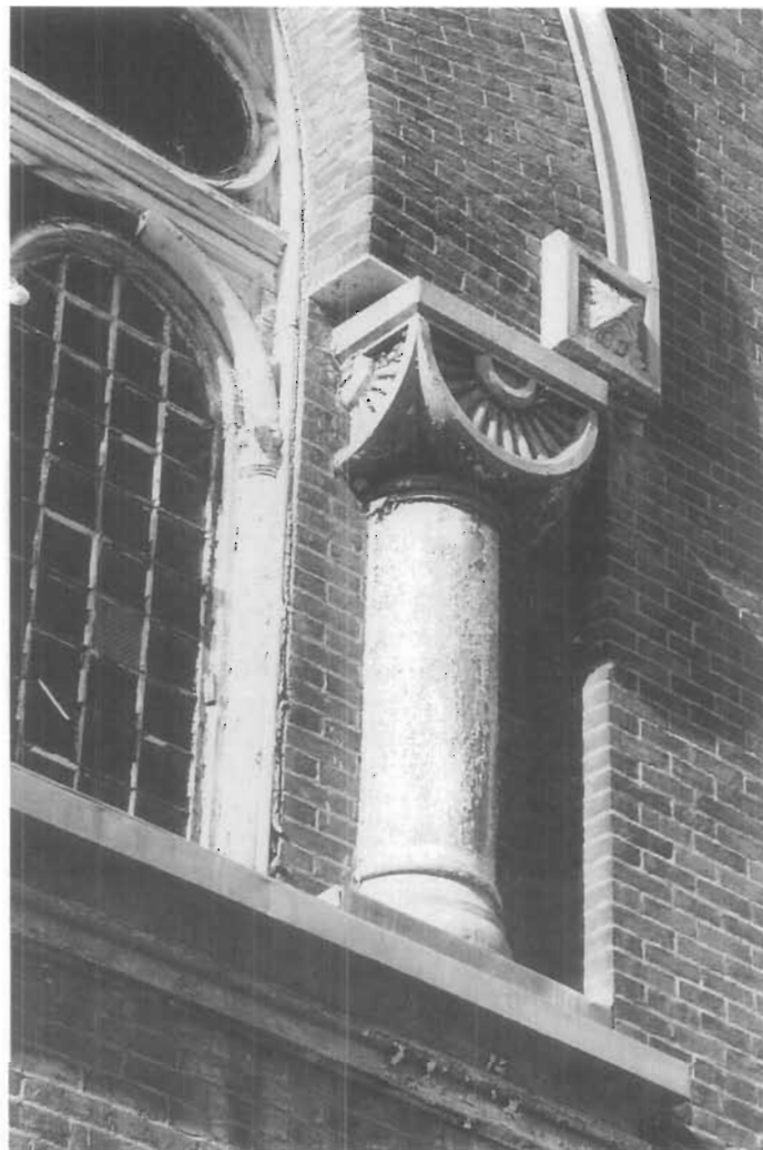
Figure 138. Zinc Deterioration and Staining. On the First Presbyterian Church in Alexandria, Virginia, the engaged columns, arch molding, corner blocks, and the sill molding are fabricated of cast zinc and galvanized sheet iron (the windows and frames are wood). The paint has deteriorated, leaving the surface of the metal bare in some places. The zinc or zinc coating on iron has oxidized. Notice the whitish corrosion stain on the brick from the zinc carbonate coating which continues to wash over the surface of the bare metal and then down over the bricks. The metalwork should be scraped down to remove all loose zinc carbonate. Joints should be caulked and/or resoldered, and repainted with a zinc chromate primer. (Baird M. Smith)
