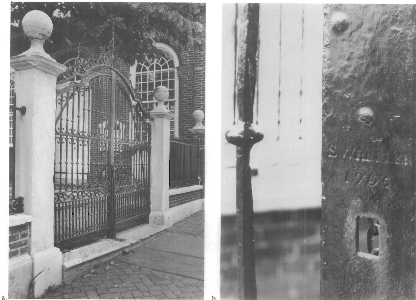
Figure 52. Wrought-iron Gates, Samuel Wheeler, blacksmith; Christ Church, 22-26 North Second Street, Philadelphia, Pennsylvania, 1727-1744; attributed to Dr. John Kearsley, builder-architect. (a) The wrought iron was heated, hammered, bent, and twisted to achieve the various parts of the design. The verticals were split and then bent to form the scrolls, rather than bent and attached to the verticals. (b) Like the balcony on Congress Hall (see figure 51), these gates are signed and dated; "S. Wheeler 1795" appears on the edge of the gate, seen only when the gates are open. (Jack E. Boucher, NAER)
