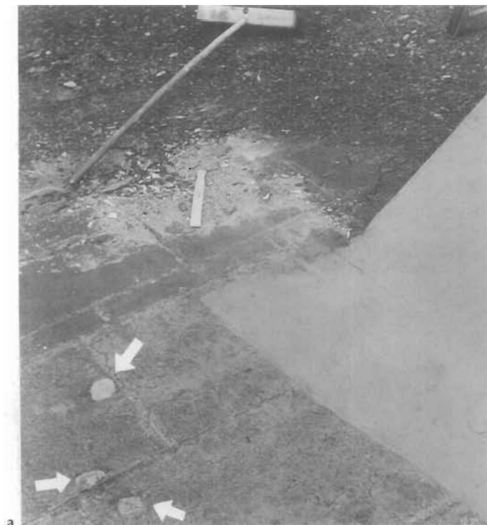
Figure 131. Salvaging a Flat Seam Terneplate Roof. (a) The roof of the Henry E. Bradford House Carriage Barn (c. 1860s) in Bennington, Vermont, had been covered with an asphalt coating (background) which obscured the true cause of the leaking roof. Once the asphalt coating was scraped from the surface (foreground left), it was noticed that the nails in the sheathing had "popped up" (light spots) and had cut through the terneplate. (b) After the asphalt coating had been scraped away and the nail holes repaired with solder (left foreground), the roof was then painted with red-lead primer (right foreground). The primed roofing was given two finish coats of iron oxide paint. (John G. Waite)
