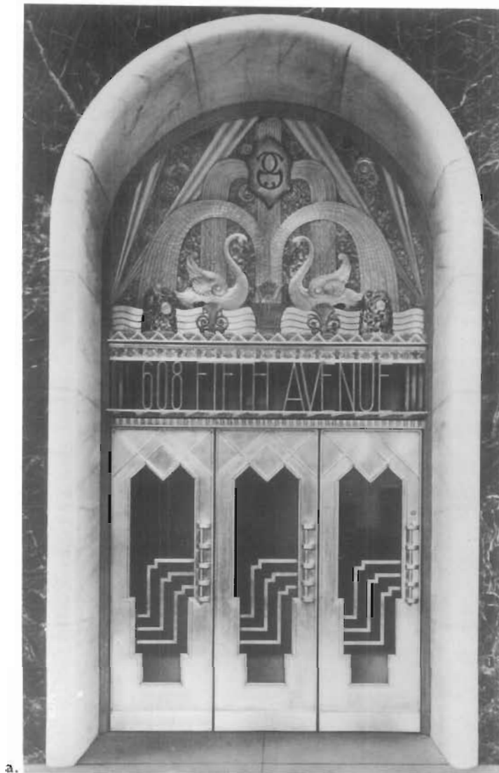
Figure 46. Nickel Silver Doors and Tympanum, Goelet Building, New York City, 1932; E. H. Faile, architect; General Bronze Corp., foundry, Long Island, New York. (a) This Art Deco-style entrance features silvery-yellow geometric doors which are almost overshadowed by the exuberant swan and fountain design in the tympanum with its array of colorful shapes. (b) The effect was achieved with a combination of copper, bronze, brass, nickel silver, and black enamel as indicated on the original drawing. When the first-floor facade was remodeled in 1966, the doors were removed and stored; the tympanum was taken to Newport, Rhode Island, to be reinstalled in a private club. (International Nickel Company)
