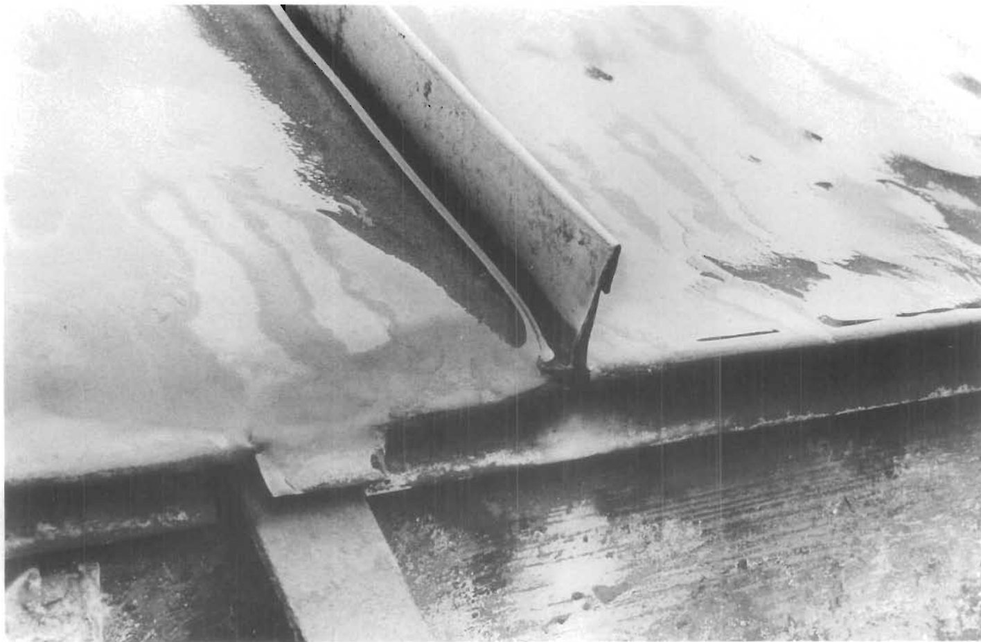
Figure 150. Erosion of Copper. This eaves detail of the 1920s copper roof on the Senate House State Historic Site in Kingston, New York, illustrates erosion of the copper at the edge of the roof caused by continued exposure to rain and snow, which scoured the roof as it flowed to the gutter. Fatigue failure has also occurred at the base of the standing seam, resulting in a tearing of the copper. This failure was caused by the lack of provision for expansion and contraction, as well as the use of bituminous roofing felts, which restricted the movement of the copper. (John G. Waite)
