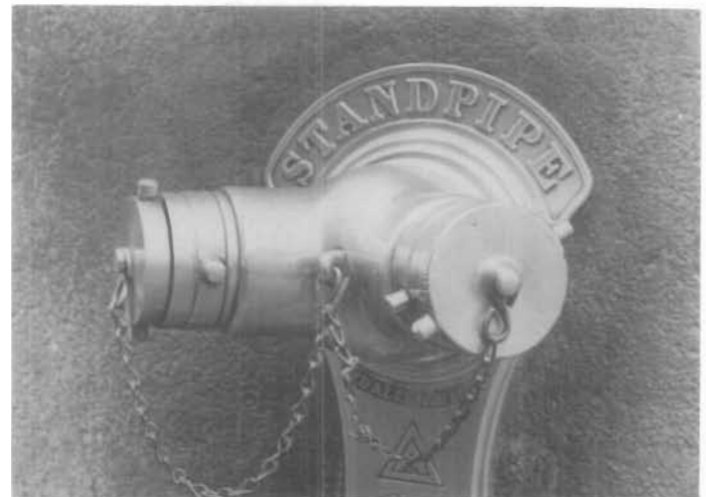
Figure 37. Brass Siamese Standpipe Connection, Rookery Building, 209 South LaSalle Street, Chicago, Illinois, 1886; Burnham and Root, architects; W. D. Allen, manufacturers. Brass fittings can be functional and very attractive when kept well polished. Even though the natural weathered dark patina on brass is protective, it is generally considered to be unsightly and great effort is expended to recapture the metallic gleam. (Margot Gayle)
