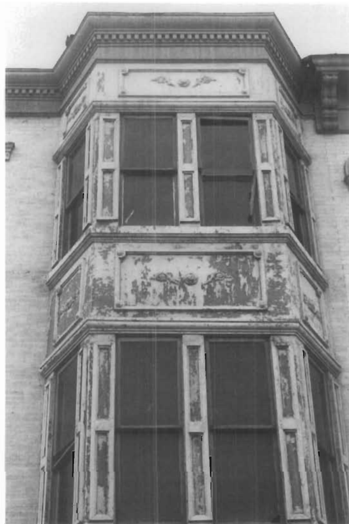
Figure 18. Galvanized Sheet Iron Bay with Applied Zinc Ornament, 608 Indiana Avenue, NW, Washington D.C. When sheet metal work is kept well painted, it is very difficult to identify it as sheet iron or steel, galvanized or tinplated. However, if the metal is not maintained, its composition becomes more obvious. Paint does not adhere well to pure zinc, or to galvanized iron or steel. When the paint peels, it usually comes off completely, including the primer, to reveal a clean metal surface. If the metal is galvanized, it will have a spangled appearance and may show some rust or rust stains from the iron base metal. If it is cast or pressed zinc, it will have a grayish-white appearance. This bay is covered with galvanized sheet iron with pure zinc ornaments on the surface. Even if well painted, a magnet test will reveal what is galvanized iron or steel (which is magnetic) and what is pure zinc (which is non-magnetic). (David W. Look)
