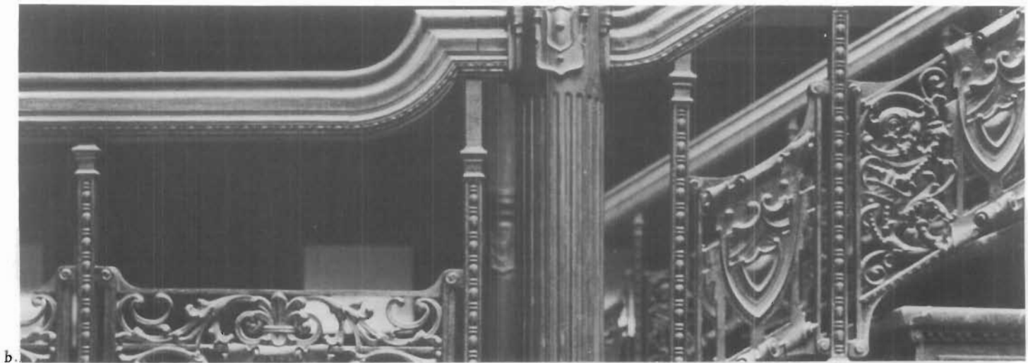
Figure 80. Light Court and Detail of Cast Iron Stairs, Bradbury Building, 304 Broadway, Los Angeles, California, 1893; George Wyman, architect; Winslow Brothers, foundry, Chicago, Illinois. (a) Built for the successful miner Louis Bradbury, this conventional masonry building gives no hint from the outside of its remarkable interior light court with its iron and glass skylight. The five-story open space has bird-cage-like elevators moving in open shafts with the machinery and counterweights exposed. (b) The elaborate openwork design of the galleries was cast in bold relief on both sides of the panels. The railings were cast in many parts and then assembled. Slender beaded balusters take the form of clawed feet where they attach to the staircase. All parts of the railing and galleries are outstanding examples of the art of sandcasting. (Becket Logan)
