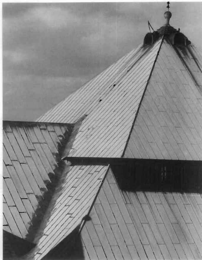
Figure 145. Galvanic Deterioration. An electrolytic reaction between the copper roof and the cast-iron roof finial and monitor window frames on the former Temple Beth Emeth, Albany, New York, built in 1887, is causing extensive deterioration of the iron. The corrosion products are staining and streaking the copper. Another area where deterioration is occurring is the valley, which has been coated with an aluminumized asphalt roofing compound. Electrolysis is occurring between the copper and aluminum (causing the less noble aluminum to corrode) and between the aluminum and cast iron of the monitor window frames (causing the less noble aluminum to corrode). (John G. Waite)
