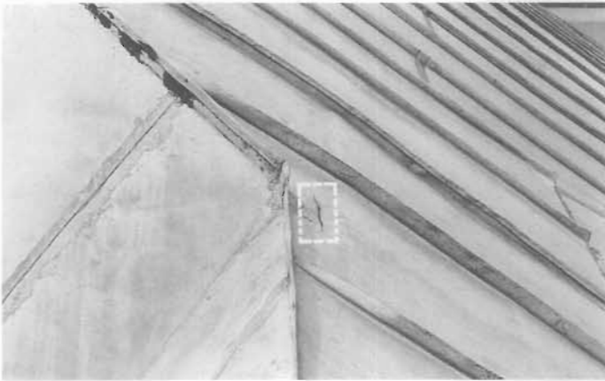
Figure 147. Fatigue Failure. Fatigue failure occurred on the copper roof installed during the 1920s on the Senate House in Kingston, New York. (a) Failure was caused by cyclical expansion and contraction of the copper without adequate provisions for it. Additionally, the copper sheet was too thin and not rigid enough to resist buckling and sagging between the too-widely-spaced roof sheathing. The use of bituminous roofing paper between the copper and sheathing also contributed to the failure; when the paper was heated by the sun, it adhered to the copper, further restricting its movement (see figure 117). (b) The drawing shows the actual roof installation and the correct procedure, which allows for expansion and contraction. (John G. Waite)
