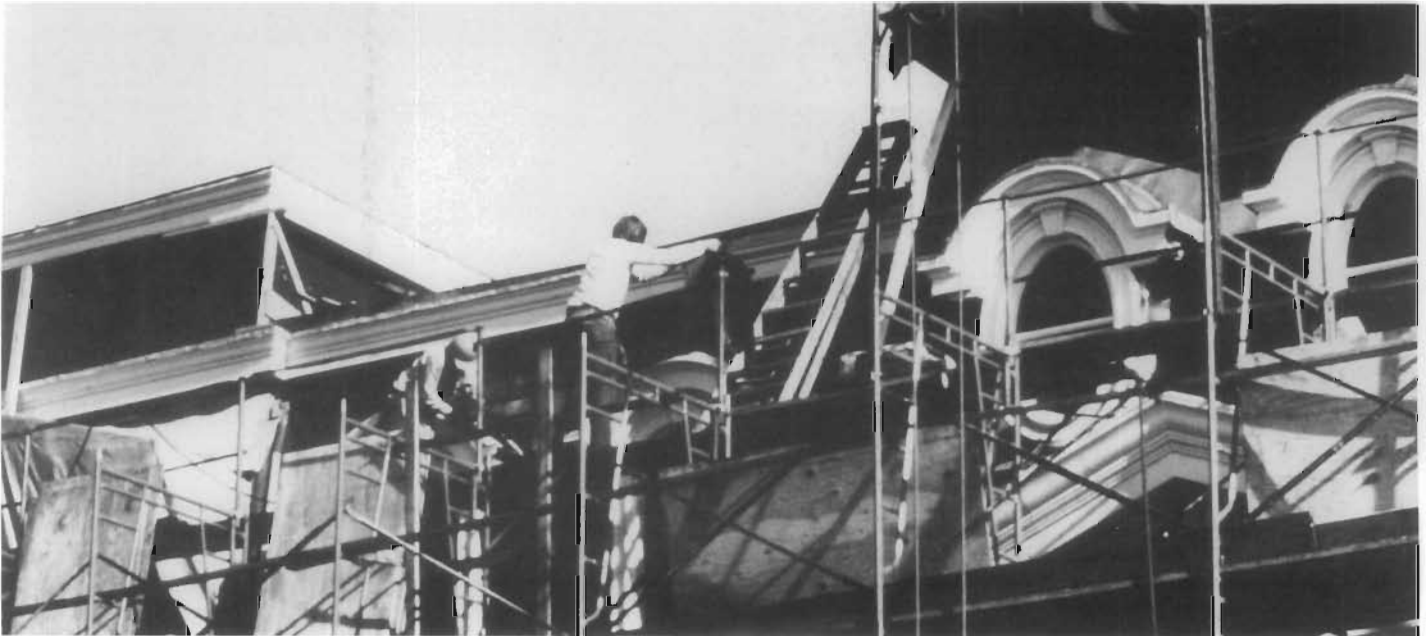
Figure 179. Use of Both Cast Aluminum and Fiberglass as Substitute Materials. After the Mansard roof and dormers of the Wilmington Grand Opera House were destroyed by fire the top floor was rebuilt, but not according to the original design. During restoration of the facade, photographs showing the original Mansard roof and dormers were found, which enabled the re-creation of the missing parts of the facade. The oval windows were cast in aluminum; but the moldings and trim, which may have originally been sheet iron, were made of reinforced polyester. (Walter Smalling, Jr.)
