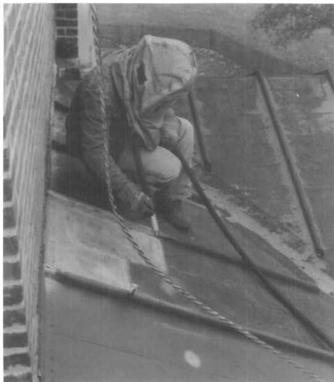
Figure 133. Abrasive Cleaning of Terneplate Roof and Replating. (a) Sections of the original terneplate roof at Lindenwald (Martin Van Buren National Historic Site) in Columbia County, New York, designed by architect Richard Upjohn in 1848, were cleaned with a low-pressure blasting of crushed walnut shells to remove accumulated paint and rust before replating with a lead/tin alloy. (b) The new terneplating was applied in localized areas (only where the original terne had been damaged by falling slates or removed because the sheet iron underneath had corroded). The new terneplating was applied where the bare iron was exposed using a soldering "copper" (a large soldering tool) fabricated for the project. After cleaning and replating, the restored roof was painted. (John G. Waite)
