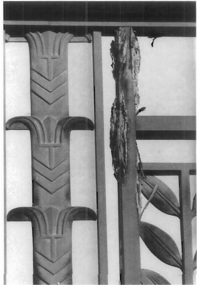
Figure 183. Exfoliation Deterioration. In Washington, D.C., at the Folger Shakespeare Library designed in 1932 by Paul Philippe Cret, the aluminum alloy balcony railing began to exfoliate in layers, similar to rusting wrought iron. The corrosion product was grayish white and lifted up from the surface as if the metal had exploded. All of the cast ornamental sections were in relatively good condition; only the straight bar stock was affected. The original specifications stated that the railing was to be an aluminum and chromium alloy. However, a recent laboratory report analyzed a four inch section cut from a sound piece of metal next to a corroded area and indicated that it was high-copper alloy (structural aluminum) fitting into the category of alloy 2017, which is not recommended for exposed outdoor use since it is not corrosion resistant. It is amazing that it lasted 47 years outdoors. All of the straight bar stock of the railing should be replaced with alloy 6063. The cast ornament could be cleaned and reused since they are obviously of more corrosion-resistant alloy and show no signs of deterioration. (David W. Look)
