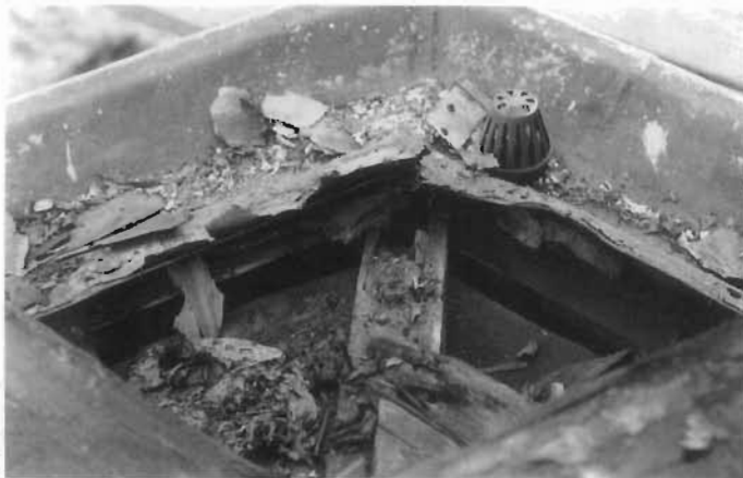
Figure 124. Successive Failure. If a metal architectural element such as a tinplate roof fails, more than just the tinplate may be destroyed. (a) Deterioration is evident in the original framing and roof sheathing of the Schuyler Mansion entrance wing in Albany, New York. The entrance wing was added to the building about 1817 and reroofed with tinplate sheets during the 19th century. The tinplate gutter liners eventually deteriorated and were replaced with copper during the 1930s. However, the tinplate roof remained and electrolysis occurred along the roof perimeter where the copper and tinplate were in contact. (b) Consequently, the tinplate was completely corroded away (as seen here) when the deteriorated roofing was removed. This resulted in major damage to the sheathing, framing, and masonry walls of the entrance. (John G. Waite)
