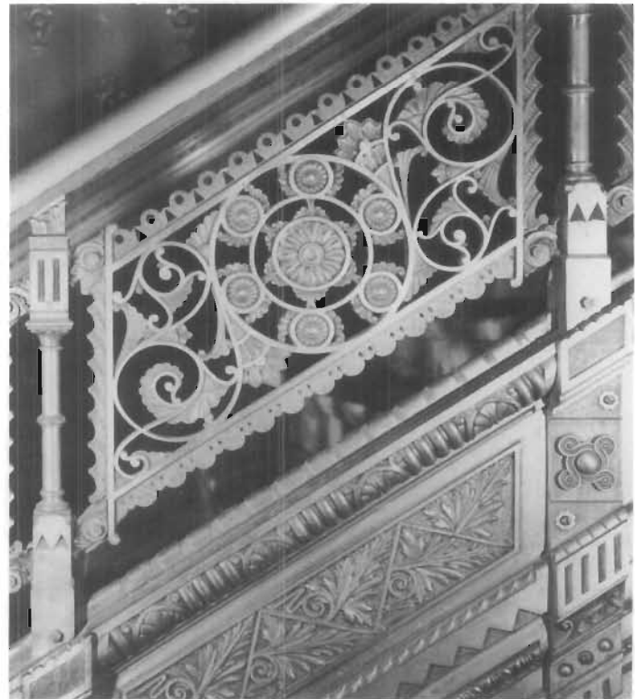
Figure 26. Copper-Plated Cast-iron Stair Railing, Christian Heurich Mansion, 1307 New Hampshire Avenue, NW, Washington, D.C., 1892–1894; John Granville Meyers, architect. This iron railing was sand cast in many pieces, and the flat areas of the design were ground smooth before the pieces were copper plated. Most of the parts were bolted together, but a few pieces of the newell post were brazed. The railing has a brass hand rail. (Jack E. Boucher, NAER)
