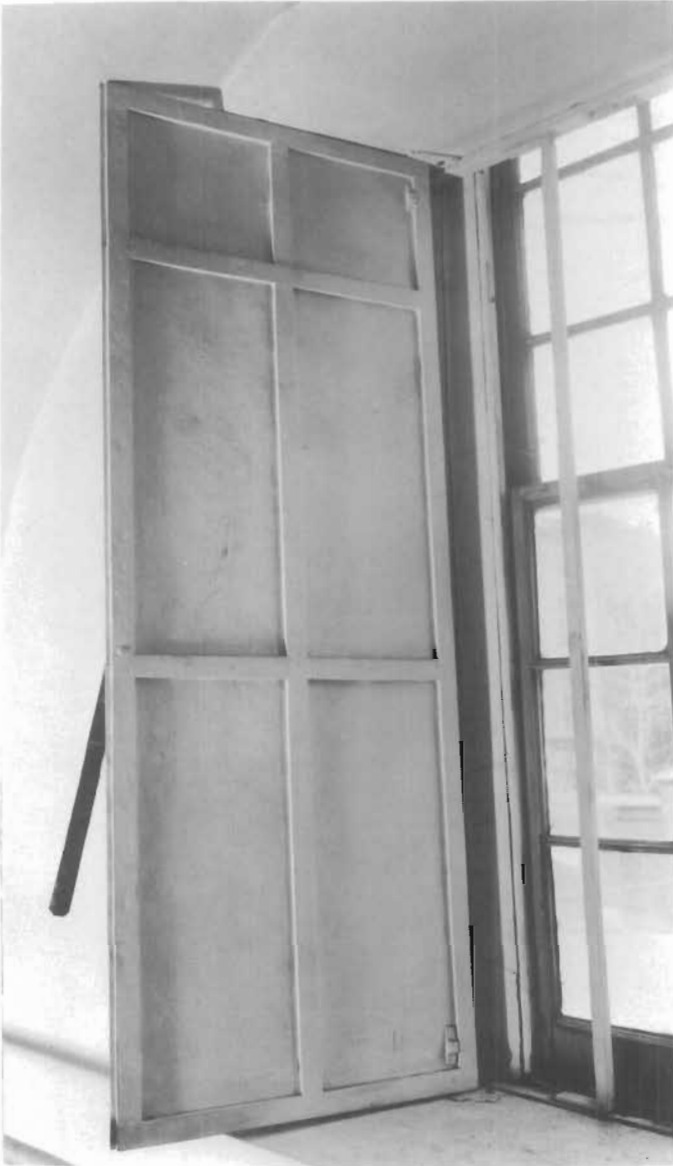
Figure 54. Wrought-iron Shutters, Arch Street Meeting House, 302-338 Arch Street, Philadelphia, Pennsylvania, 1803-1804; Owen Biddle, architect and master builder. The shutter is on the window of the "fireproof" vault used to store records. The iron shutter has a frame of hand-forged rectangular bars to which a series of rolled sheets was riveted. (George Eisenman)
