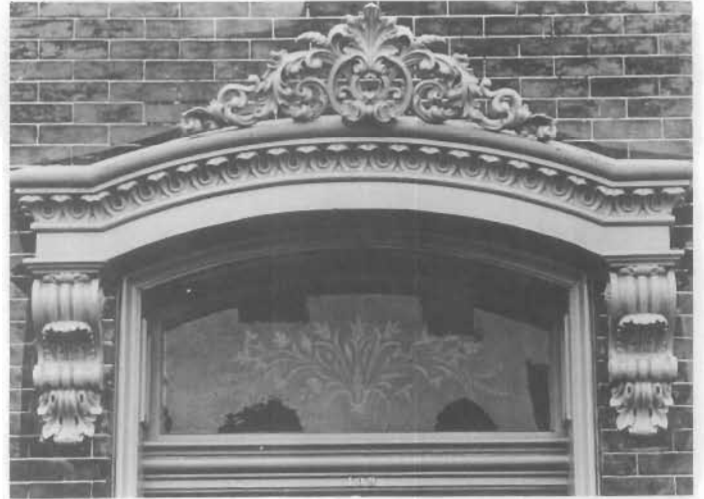
Figure 84. Cast-iron Lintel, Ben Whitmire House, 109 Jackson Street, Trenton, New Jersey, 1872. The scrollwork of the foliated lintel is clearly of cast metal; execution of such a design in stone would be almost impossible. This house also has window lintels and sills of iron, all of which were probably cast at Bottom and Tiffany's Foundry in Trenton. They were often painted stone colors with sand added for the correct texture. Residences, commercial buildings, institutions, and even industrial buildings incorporated ornate lintels and sills in their design. (Ben Whitmire)
