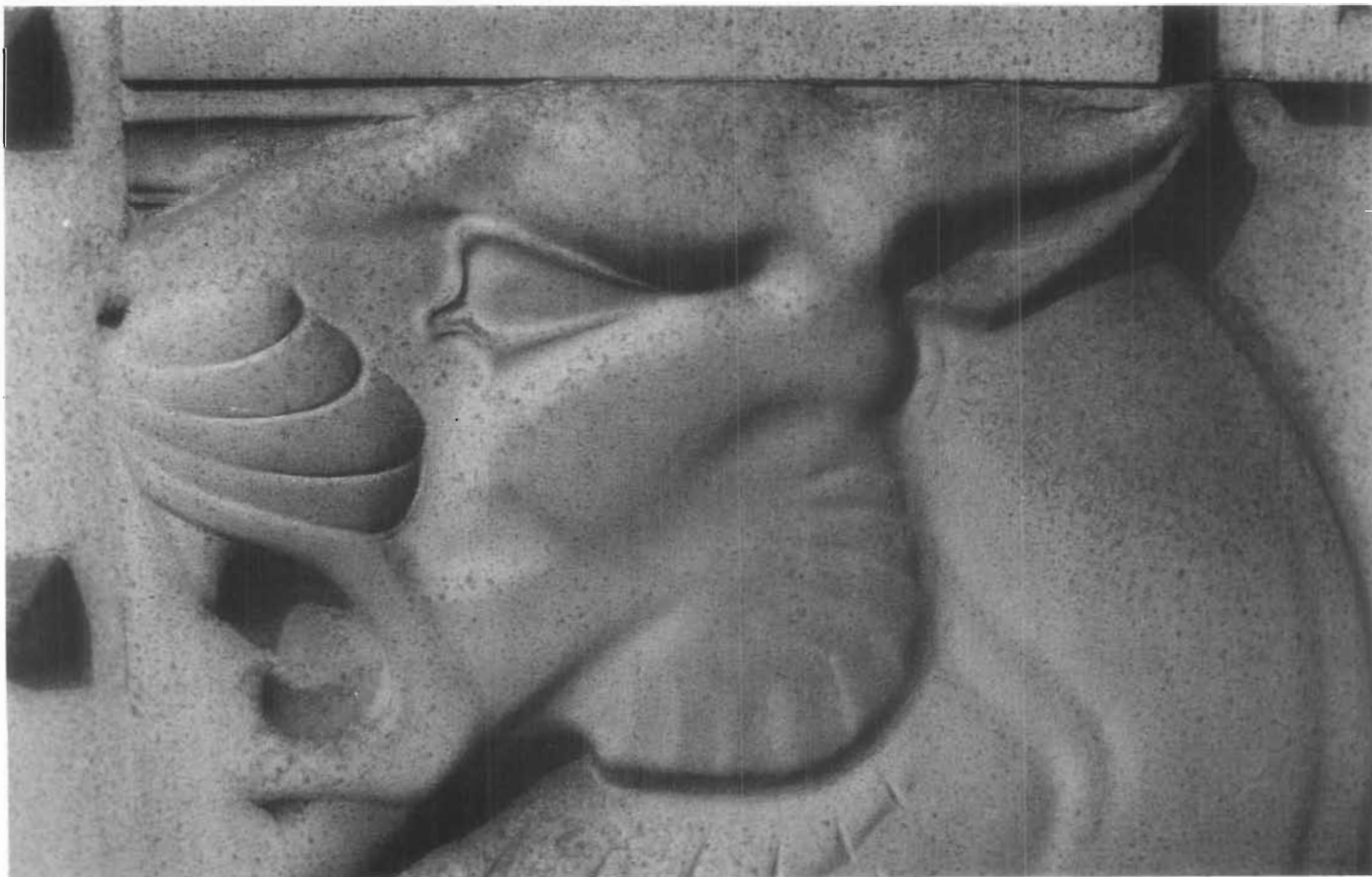
Figure 181. Corrosion and Pitting of Aluminum. Designed by Carl Paul Jennewein, these cast-aluminum doors on the U.S. Justice Building in Washington, D.C., are pitted (see figure 114). Aluminum corrosion is white; however, surface dirt, grime, and pollution have collected on the corrosion products, forming small dark bumps. The pits are actually beneath the bumps and were formed as surface metal oxidized. Pitting is caused by a difference in potential of two or more points on the surface of the same metal and a local breakdown of the protective oxide film. It is encouraged by foreign particles, such as dirt and chlorides which hold moisture next to the surface. (David W. Look)
