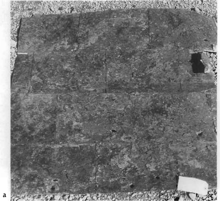
Figure 129. Corrosion Failure of Terneplate Roofing. Hyde Hall, built between 1817 and 1833, near Cooperstown, New York, was roofed with flat-seam terneplate. (a) The plates have deteriorated because of a lack of proper maintenance. Unfortunately, the exposed (top) surface of the terneplate was painted with asphalt coating, which accelerated the corrosion of the roofing. (b) The terneplate also corroded from the underside. When installed, the terneplate was not painted on the underside as it should have been. Condensation formed on the unprotected bottom side of the metal roof and could not evaporate, an ideal situation for corrosion. (John G. Waite)
