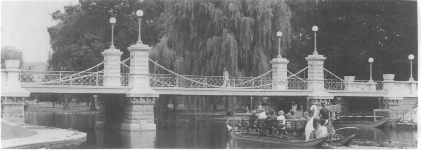
Figure 61. Suspension Bridge, Public Garden, Boston, Massachusetts, 1867; Elemens Herschel and William Preston, engineers. Popular among Bostonians, this small suspension bridge originally consisted of plank flooring hung from chains made of flat wrought-iron links. In 1921 the bridge's deteriorated wood was replaced with steel beams; the bridge was reinforced in 1975 with more steel and concrete. Although the deck has been replaced, the masonry piers and the chains hung between them are still largely original. (Carleton Knight, III)
