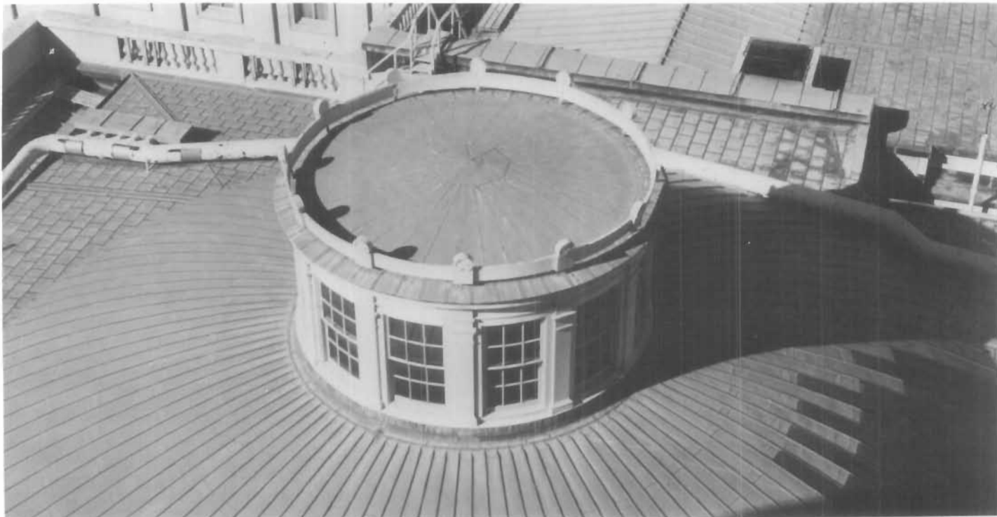
Figure 19. Copper Roof, Old Senate Chamber, United States Capitol, 1819; Benjamin H. Labrobe, architect. After the British burned the Capitol in 1814, the entire structure was rebuilt, including a new copper roof. Little is known about the roofing installed in 1819 since it was removed in 1900. It was probably all flat seams because the machine for forming standing seam roofing was not invented until about the time of the Civil War. When the surfaces were reroofed in 1975, every effort was made to duplicate the 1900 roofing patterns, configuration, and size of sheets. Sheet copper can be shaped to cover many types of curved surfaces. The dome has standing seams while the cupola and the area around the dome, which is flatter, have flat seams. (Charles Parrott)
