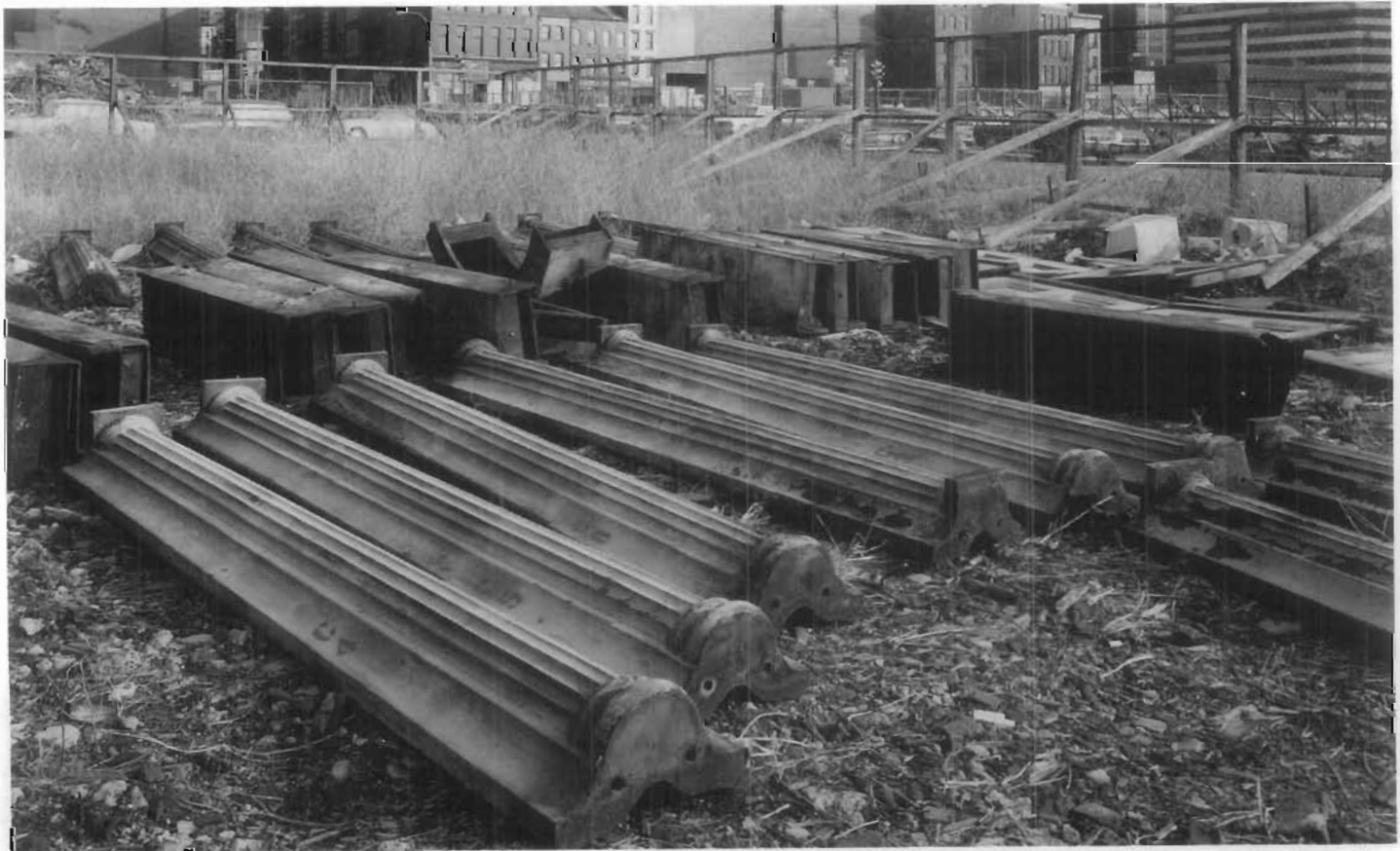
Figure 168. Dismantled Cast-Iron Facades. The Edgar Laing Stores in New York City were erected by James Bogardus in 1849 and had one of the earliest cast-iron facades. The building was demolished in 1971 for an urban renewal project, but its cast-iron facade was carefully dismantled so it could be reerected on another site at a later date. Unfortunately, while the components were in storage, most of them were stolen and apparently sold for scrap. Dismantling of a building should be considered a measure of last resort, to be attempted after all other efforts to save a building in situ have failed. (Jack E. Boucher)
