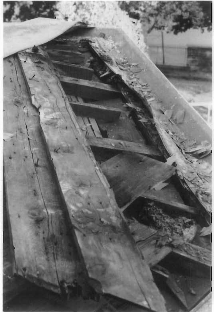
Figure 124. Successive Failure. If a metal architectural element such as a tinplate roof fails, more than just the tinplate may be destroyed. (a) Deterioration is evident in the original framing and roof sheathing of the Schuyler Mansion entrance wing in Albany, New York. The entrance wing was added to the building about 1817 and reroofed with tinplate sheets during the 19th century. The tinplate gutter liners eventually deteriorated and were replaced with copper during the 1930s. However, the tinplate roof remained and electrolysis occurred along the roof perimeter where the copper and tinplate were in contact. (b) Consequently, the tinplate was completely corroded away (as seen here) when the deteriorated roofing was removed. This resulted in major damage to the sheathing, framing, and masonry walls of the entrance. (John G. Waite)
