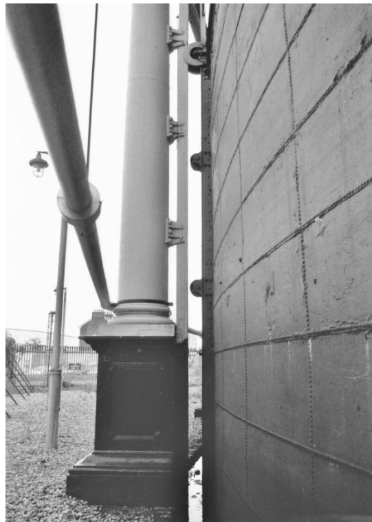
Figs. 4a and 4b. Bethnal Green No. 2, cast-iron column base at edge of the tank (MTT).
