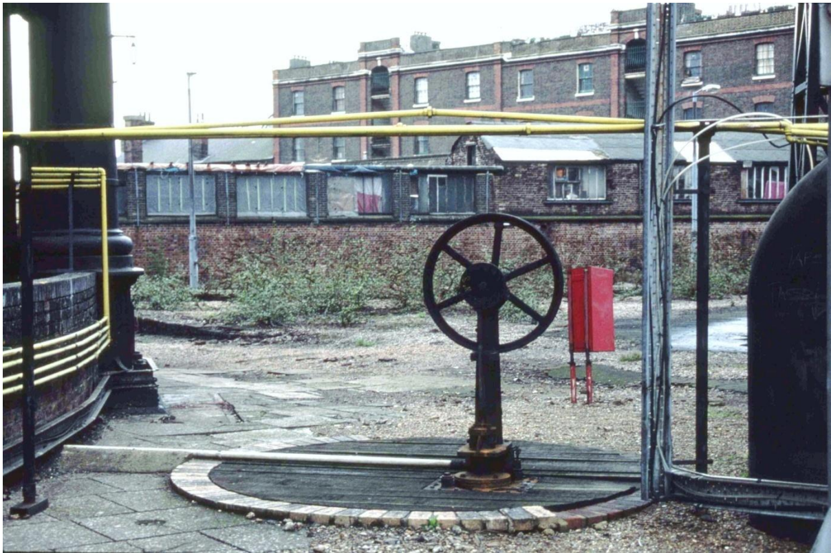
Fig. 6. Dry well and pump at No. 8 Gasholder, view from west (MTT). (The photo also shows a 20 th -century wall that had been built around the gasholder tank).
