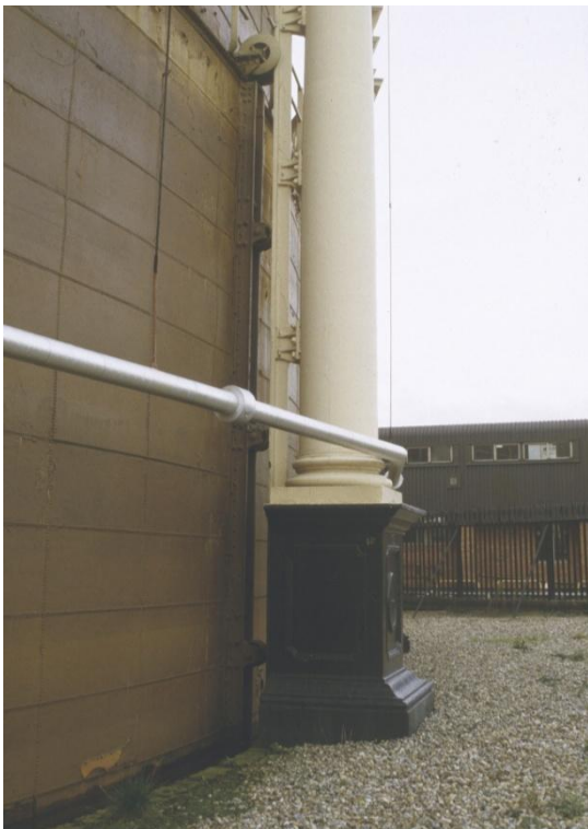
Figs. 4a and 4b. Bethnal Green No. 2, cast-iron column base at edge of the tank (MTT).
