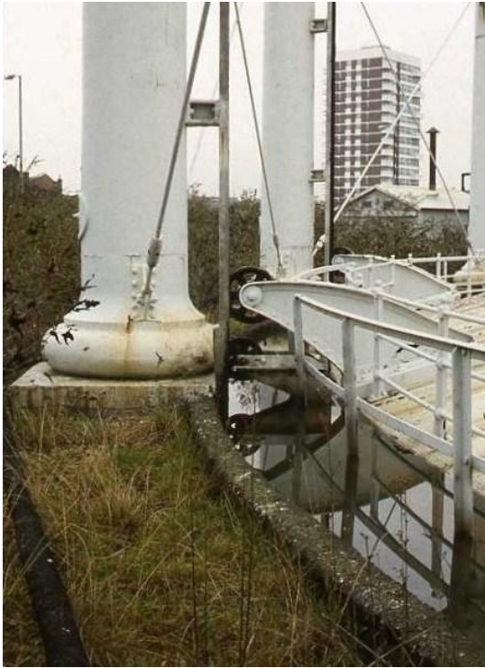
Fig 3a (above). Carriages and guide wheels at Stepney No. 2 (MTT).
