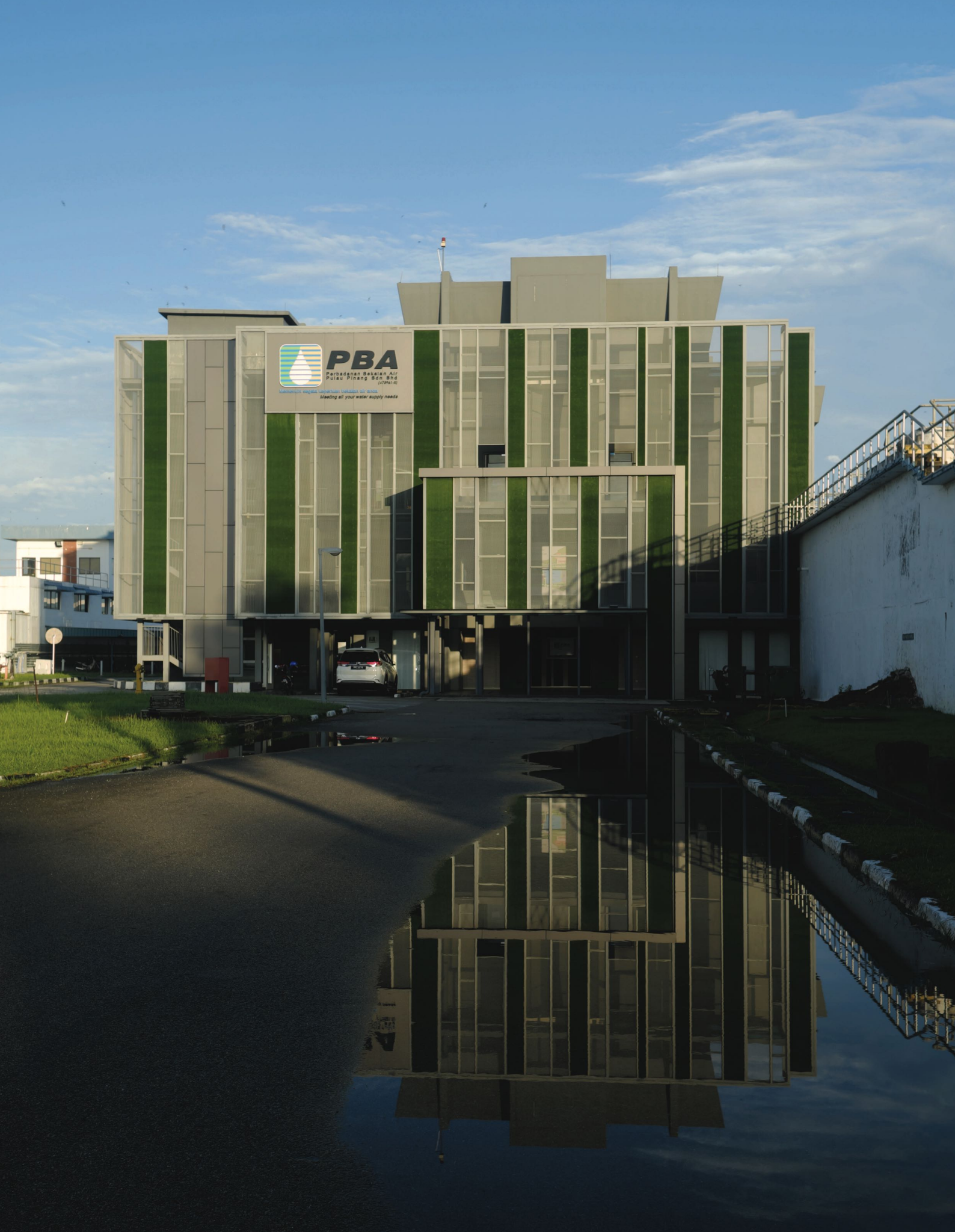
Sungai Dua New Office Complex
