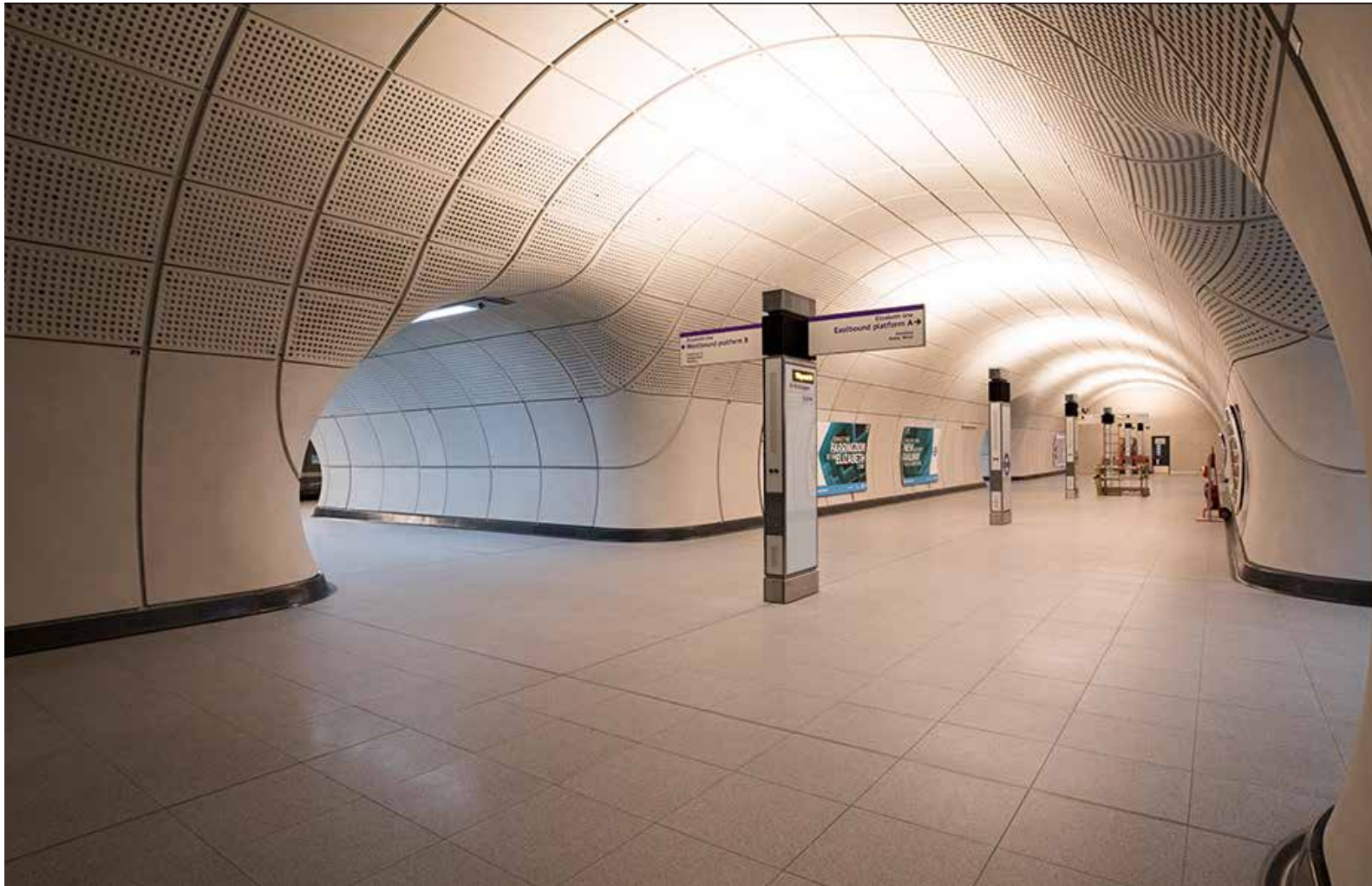
Elizabeth Line Farringdon Station. Courtesy of BAM Ferrovial Kier JV
