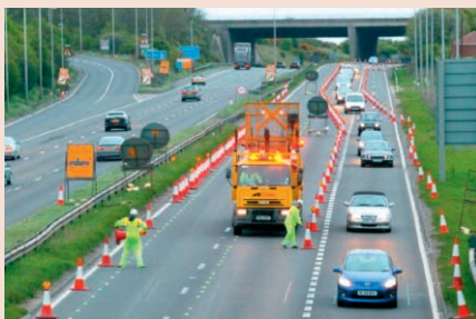
A-one+ has been reducing carriageway crossings
