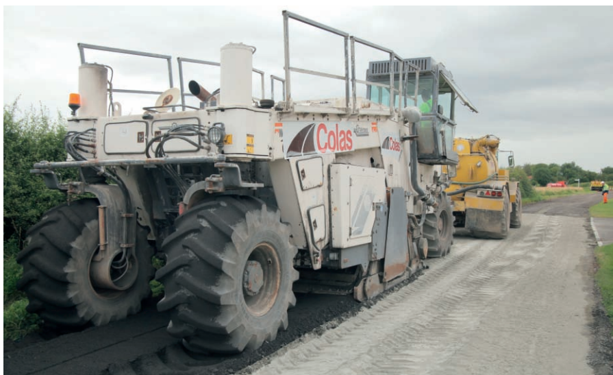
Deep recycling at Bushton: A mix of PFA cement binder creates a more flexible pavement
