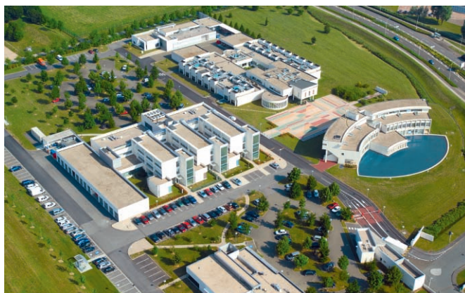
Campus for Science and Techniques, the Colas research facility in Paris
