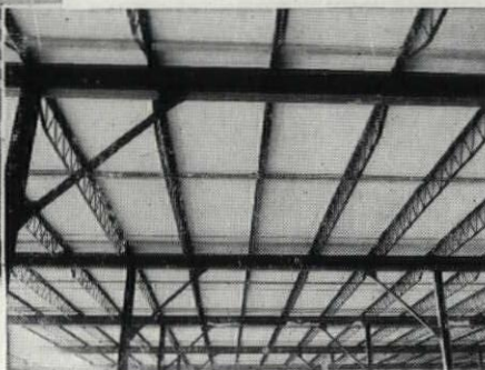
Light steel framing for 53,760 sq. ft. of Cemesto for Watson Terminal Warehouse Co., Youngstown, O.
