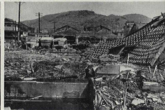
4 MILES: due to skip effects of blast, some buildings were damaged as far out as eight miles. Wood had poorest resistance.
