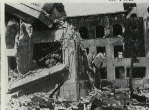
1300 FT.: reinforced concrete school suffered roof collapse when columns on blast side gave way. It was completely burned.
