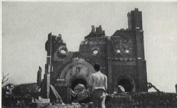
2000 FT.: weakness of load-bearing brick wall is proved in this church which had only front wall standing after blast swept through.
