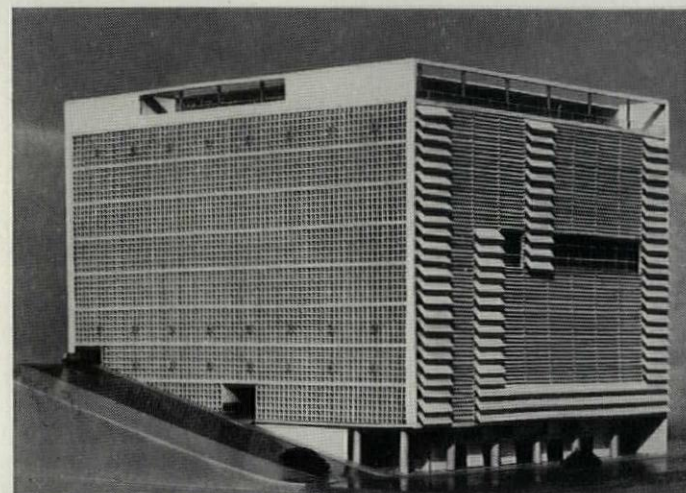
1949—Publishing building in Rio (right). Since the plant is used for early morning work, the east face (on hillside) is equipped with sunbreaks as well as the north.
