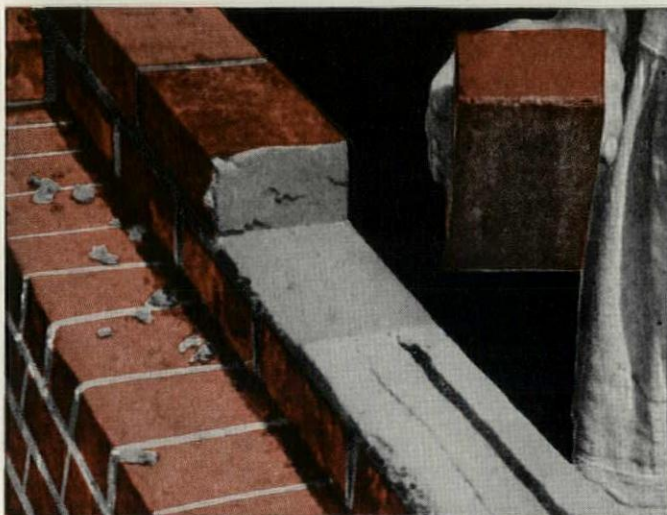
A good bond was not secured here because the brick on which the mortar was spread had sucked the mortar dry, before the brick was laid.
