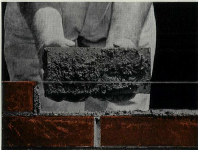
A good bond was secured here because the mortar was not sucked dry too fast.
