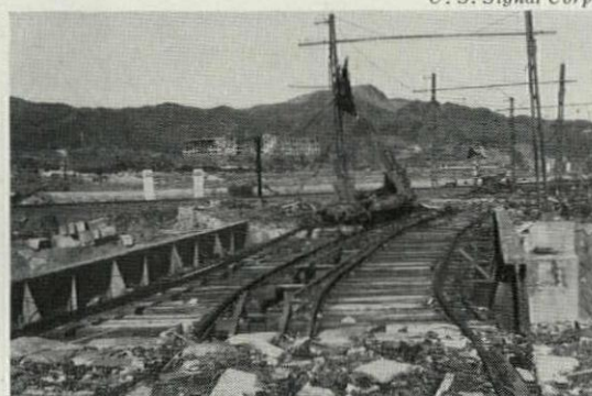
840 FT.: from "ground zero" (point beneath explosion) terrific blast moved bridge 3 ft., bending rails but leaving steel poles standing.
