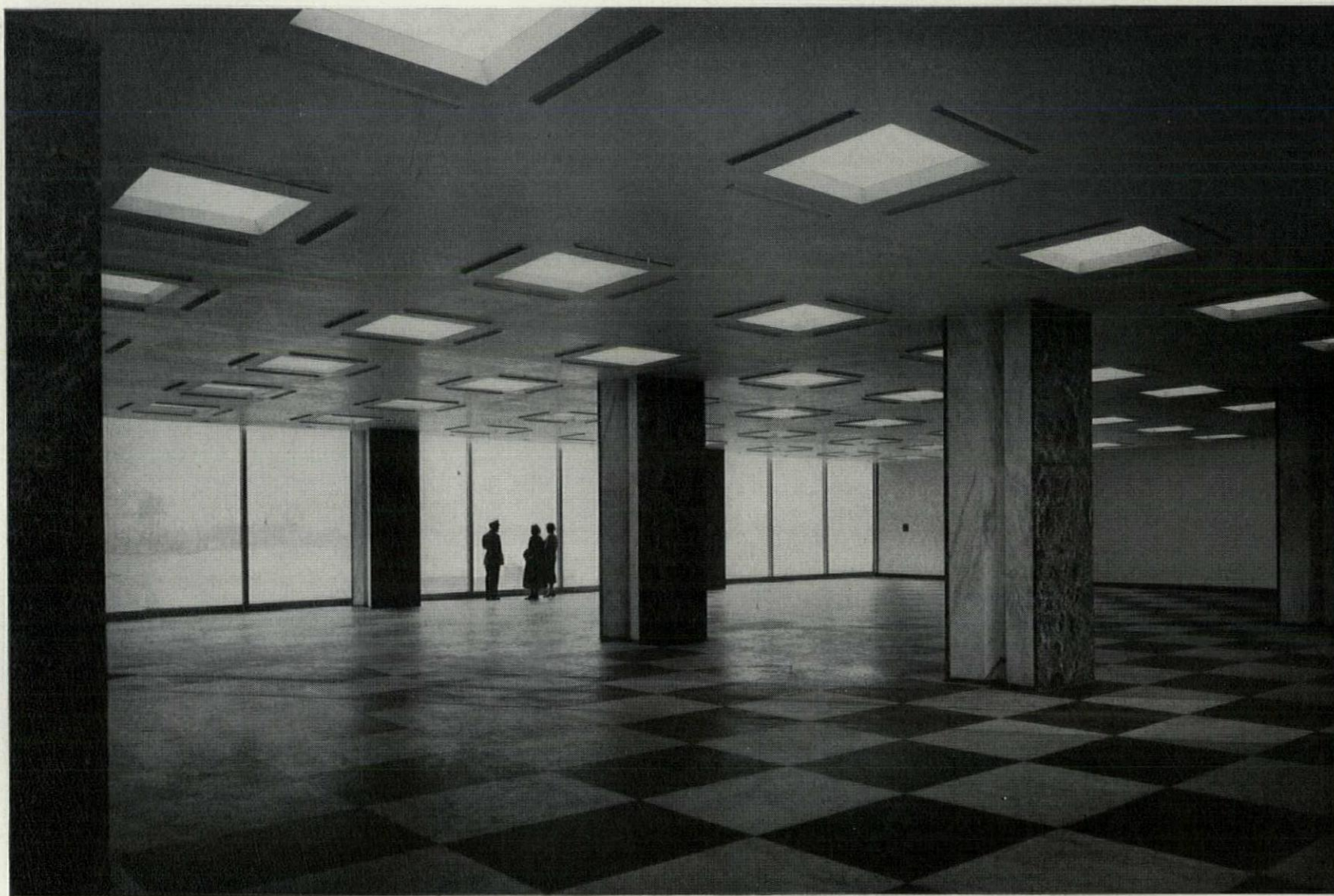
Secretariat's lobby has cove lighting that bounces fluorescent light from concealed tubes. Rectangular slots are air grilles.
