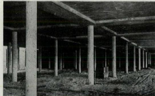
Simple lumber bracing devices will keep the fiber forms aligned as the concrete is poured into them.
