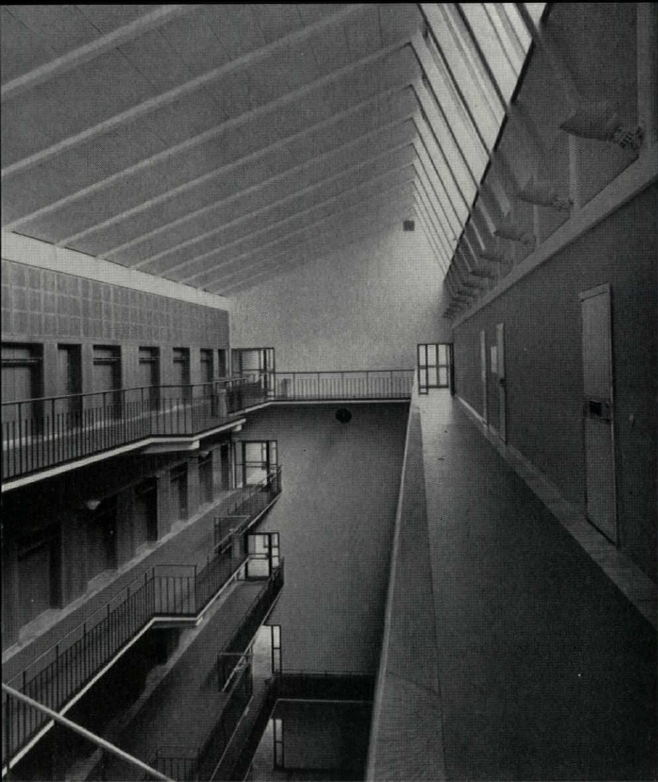
Eastern sunlight pours into the central well through a double glass skylight, warming the building's heart and accenting the airy structure of corridor balconies. (photo above) The steeply pitched ceiling of white acoustical tile absorbs sound and serves as a reflector for both natural and artificial light. Panels between indirect lighting fixtures on the east wall are new, flush-type radiators with welded vertical tubes. Boldly sculptured wall opposite has oak panelling, (slotted for acoustics) and recesses for coats set between closets for storage of teaching materials.
