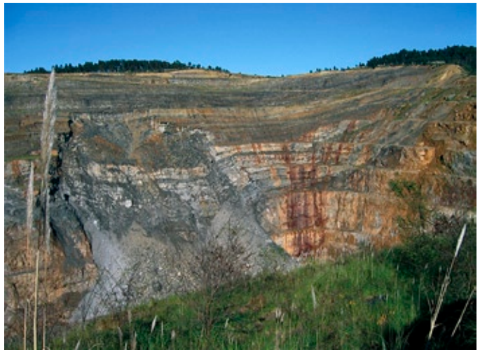
Open-pit of the Reocín mine (Torrelavega, Santander). The landslide affecting the left slope forced the exploitation to stop a few months before its planned closure in 2003.
