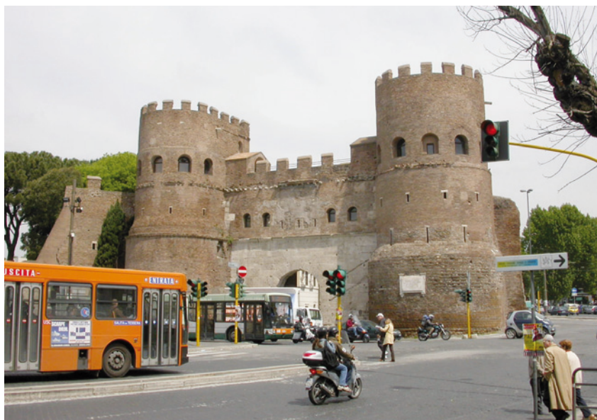
Figure 22. The well-preserved walls of Aurelian are a recurring feature of the urban image of present-day Rome. The present appearance of the walls and gates, such as here at Porta San Paolo, is the result of a number of later re-fortifications.
