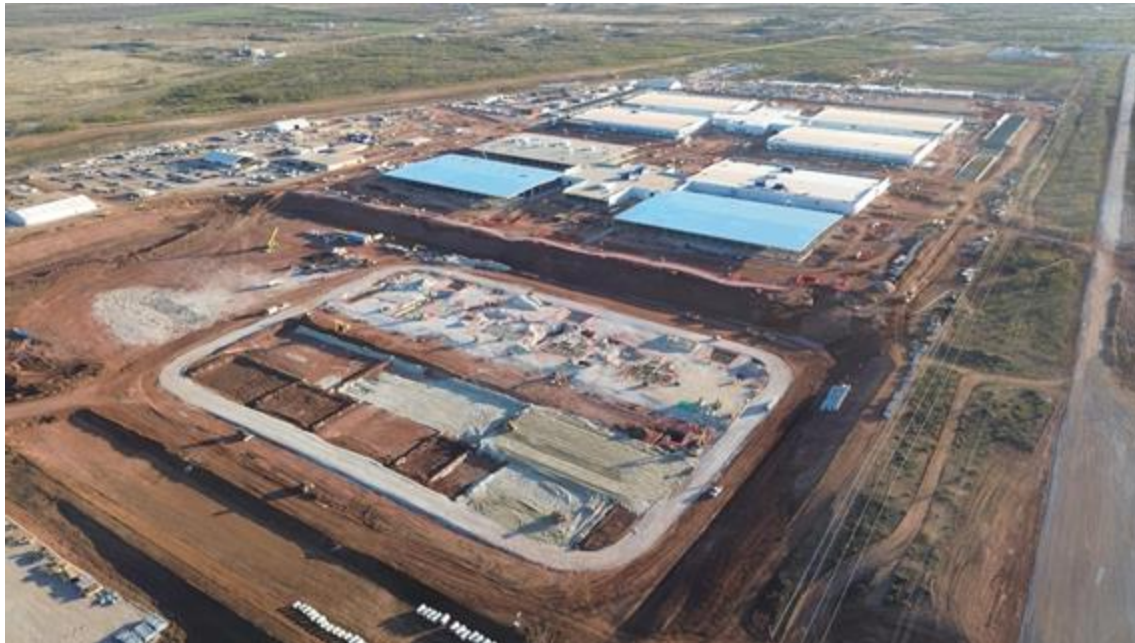
1.2 GW Lancium Clean Campus under construction in Abilene, Texas
