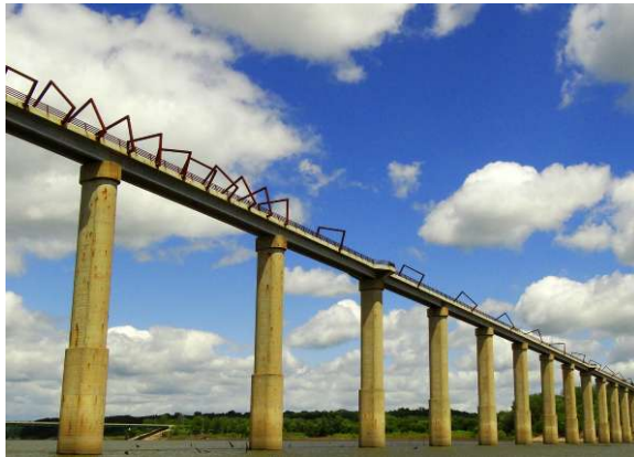
High Trestle Trail Bridge
