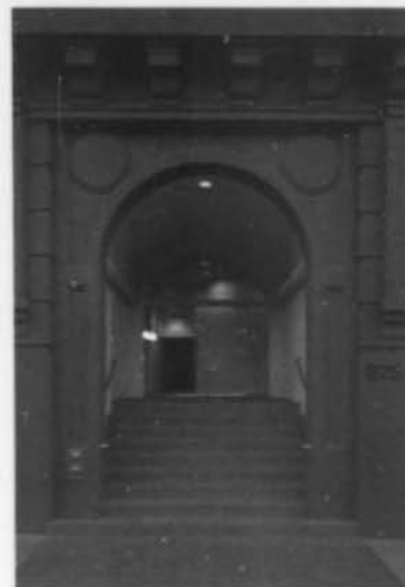
Above: New doorway and lobby inserted into entrance of the industrial building.
